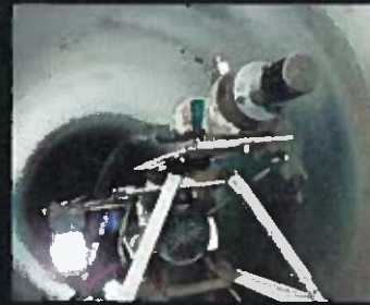
EcoCast spin casting sled begins the application process
