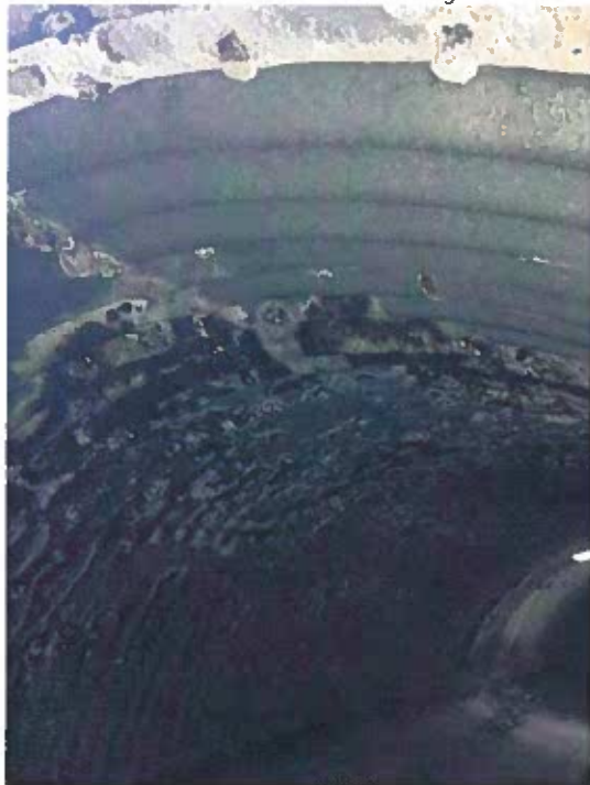
Figure 1 Corrosion Along Little Shooks Run Pipe under North Institute
