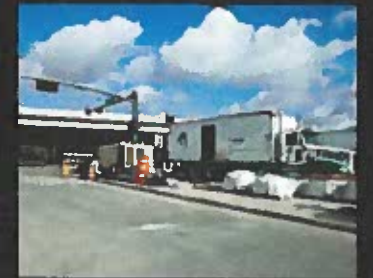
DOT projects: highways and bridge overpasses
