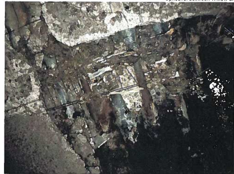
Figure 4 Upheaval Between Willow and Hancock, Plate Arch and Concrete Flood Heaved but Intact
