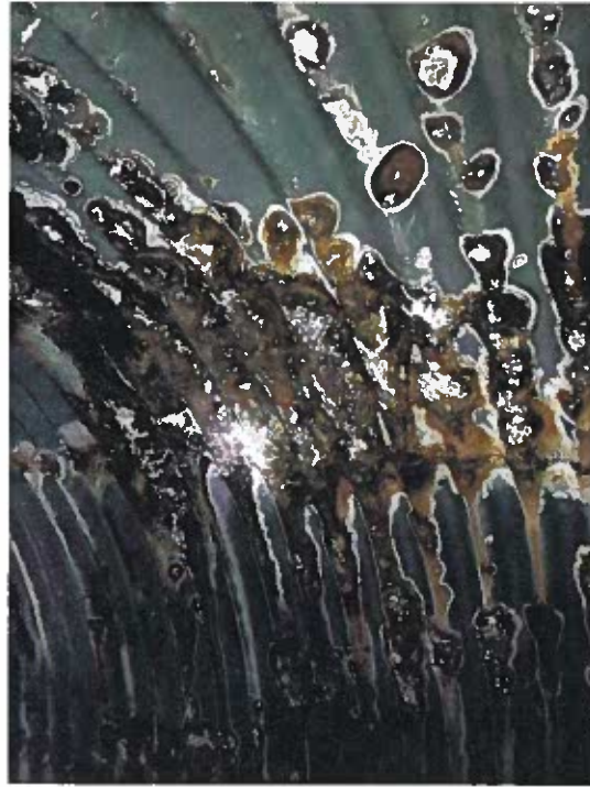
Figure 1 Corrosion Along Little Shooks Run Pipe under North Institute
