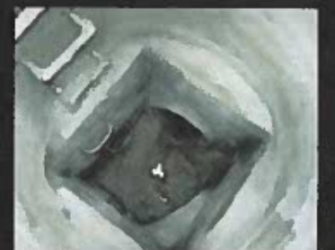
Manholes and wet wells
