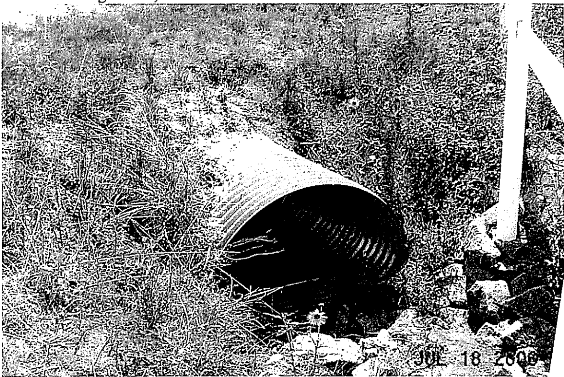
Dodge Circle, 54" w x 38" h CMP Inlet, bent.
