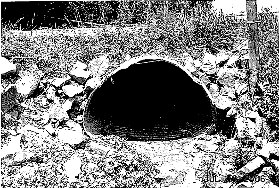
Dodge Circle, 62" w x 33" h CMP Outlet, bent.
