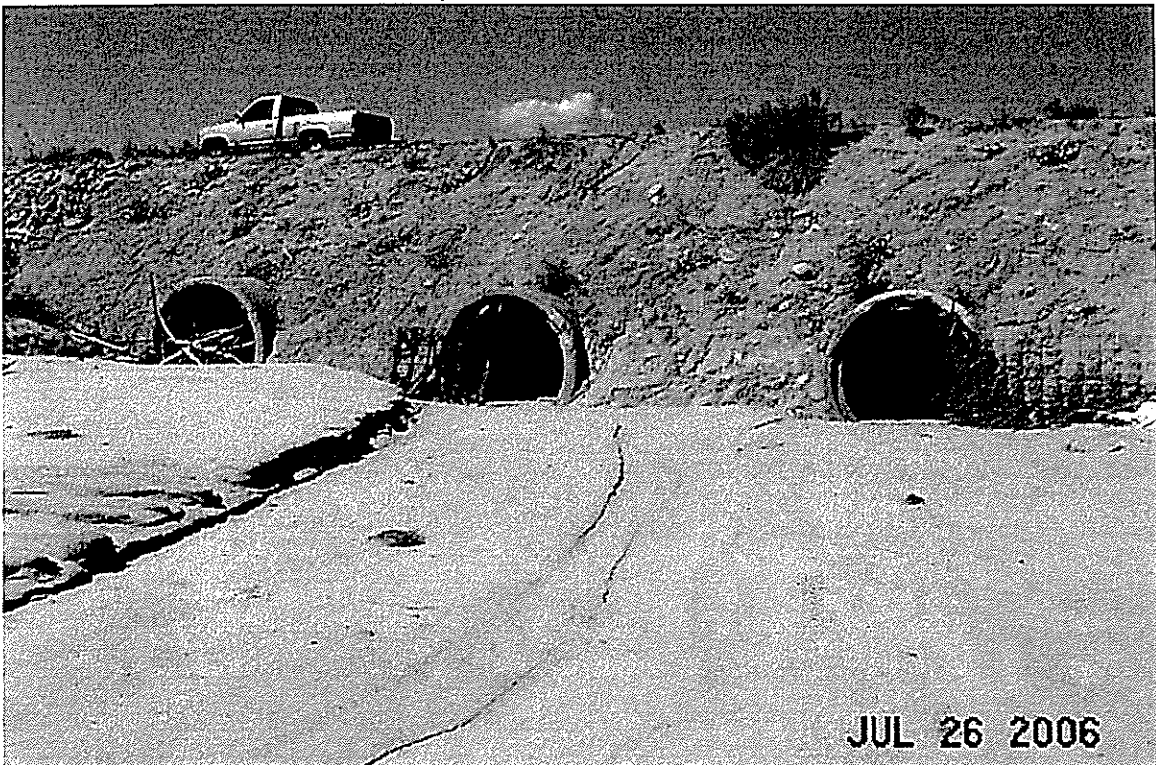
Franceville Coal Mine Road, Three 60" RCPs Inlet.
