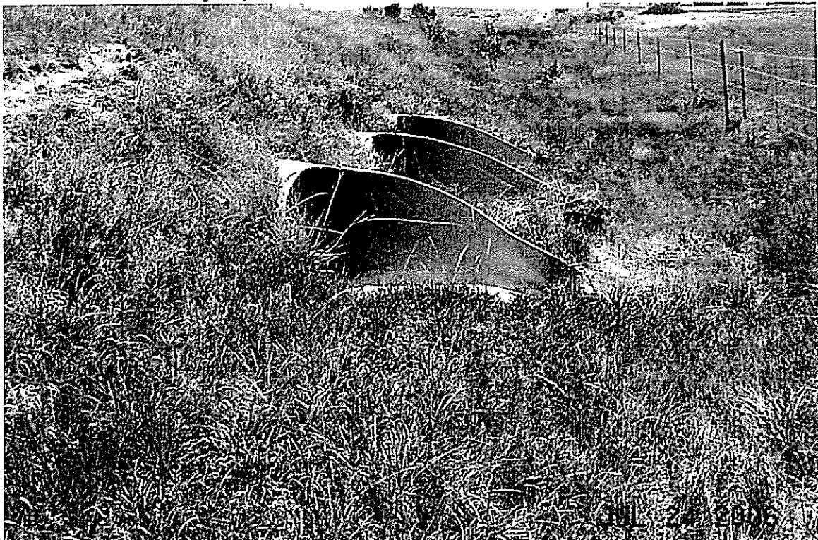
State Hwy 94, Three 36" CMPs Inlet.
