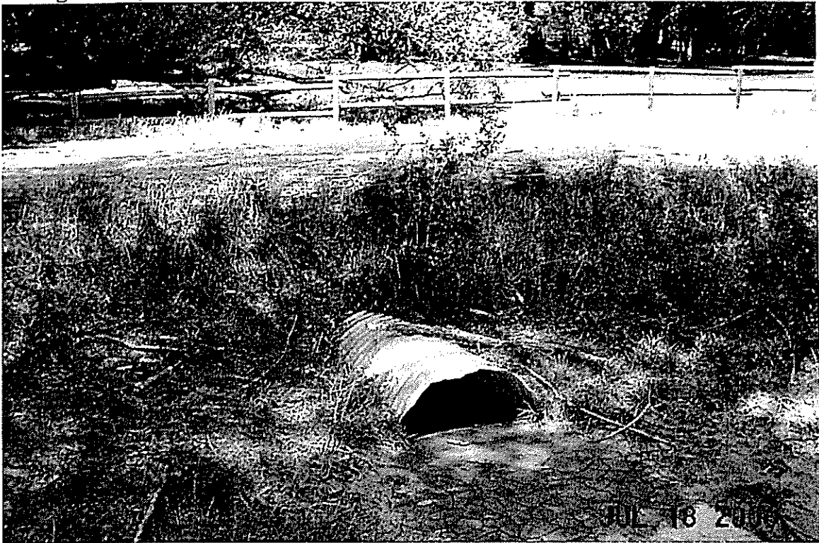
Dodge Circle, 24" CMP Outlet, bent at outlet.
