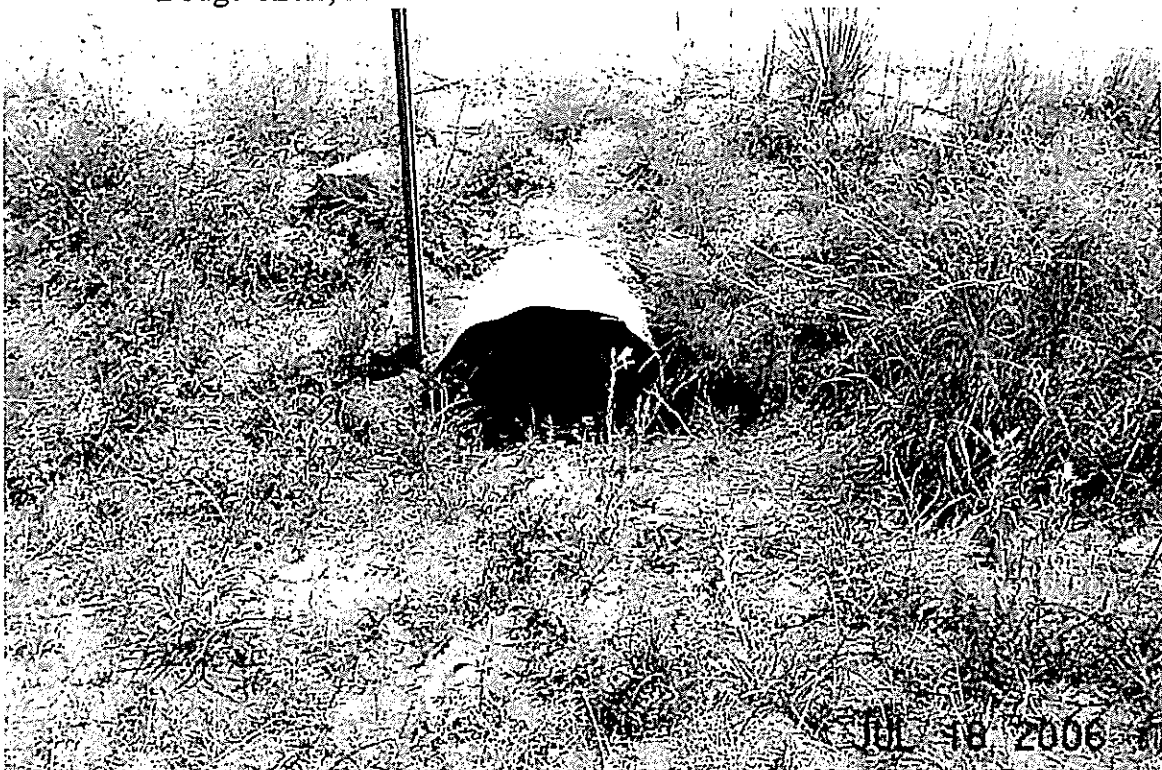
Dodge Circle, 30"w x 18" h CMP Inlet, bent.
