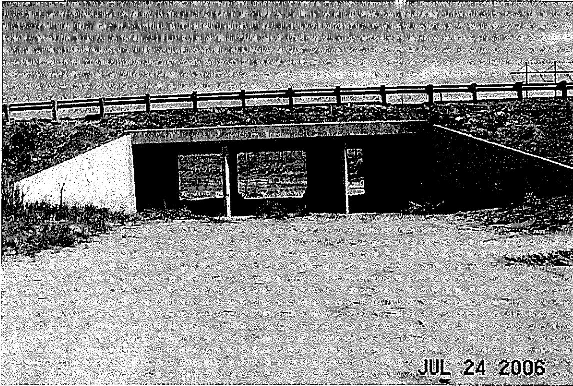
State Hwy 94, 37'3"w x 10'h Concrete Bridge Outlet.
