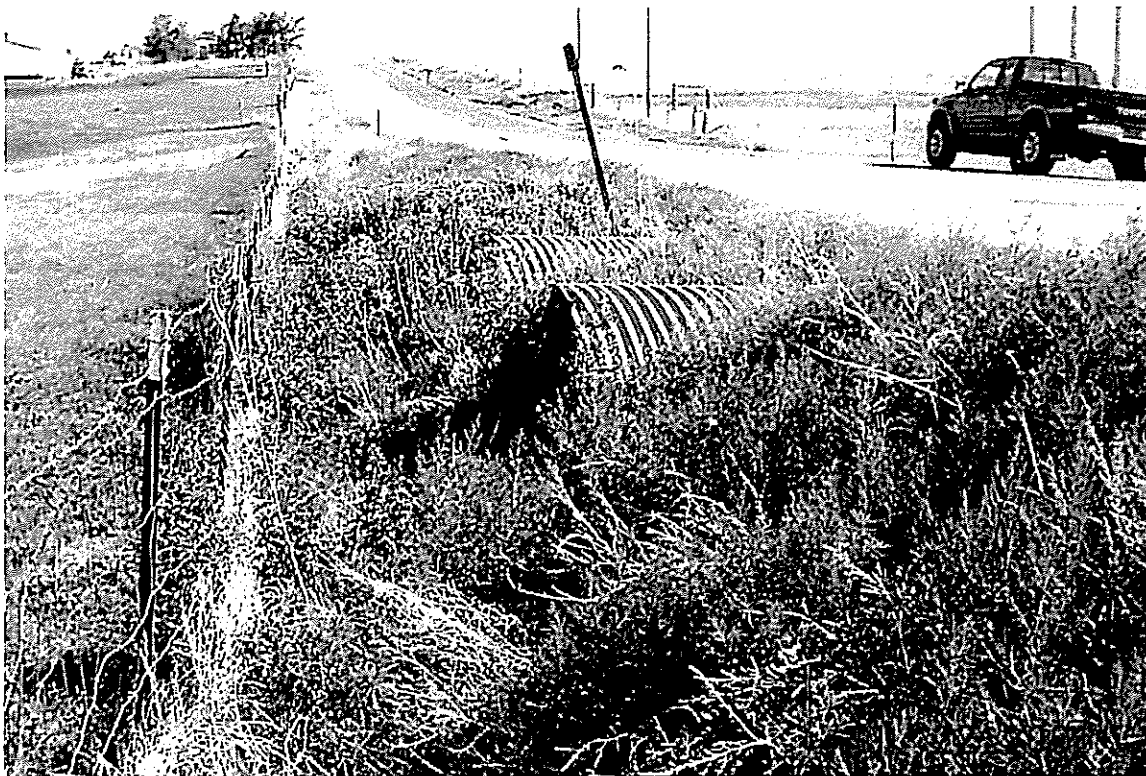
Meridian Road, Two 64" w x 42" h CMPs Inlet. Bent.
