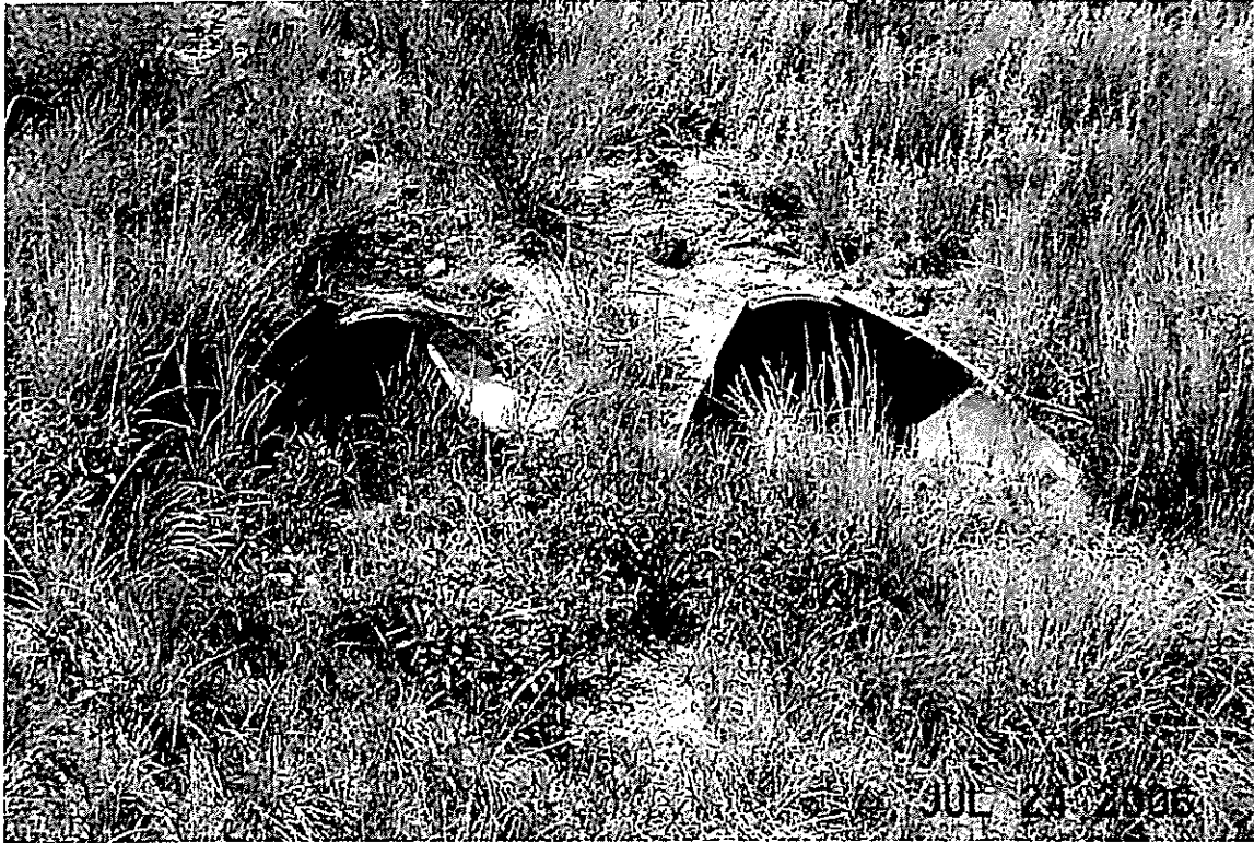
State Hwy 94, Two 24" CMPs Outlet, bent.
