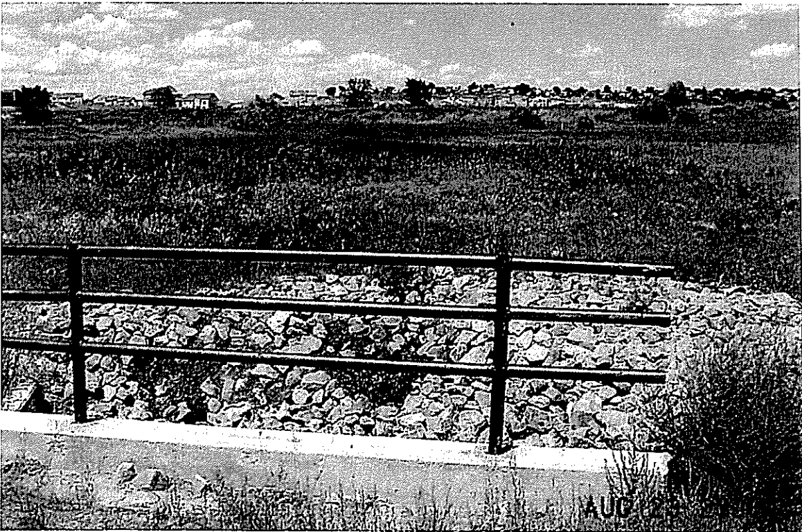
C & S Road, 12' w x 6' h concrete box culvert inlet channel. 6
