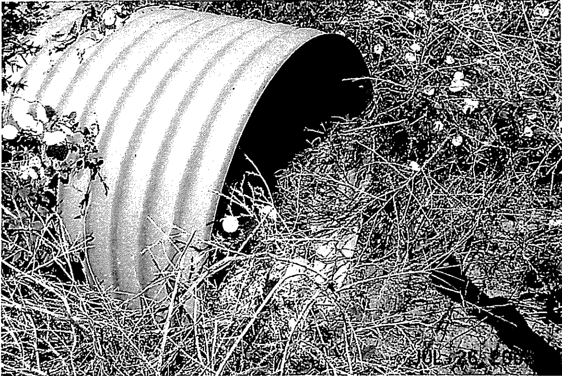
Franceville Coal Mine Road, 30" CMP Inlet.
