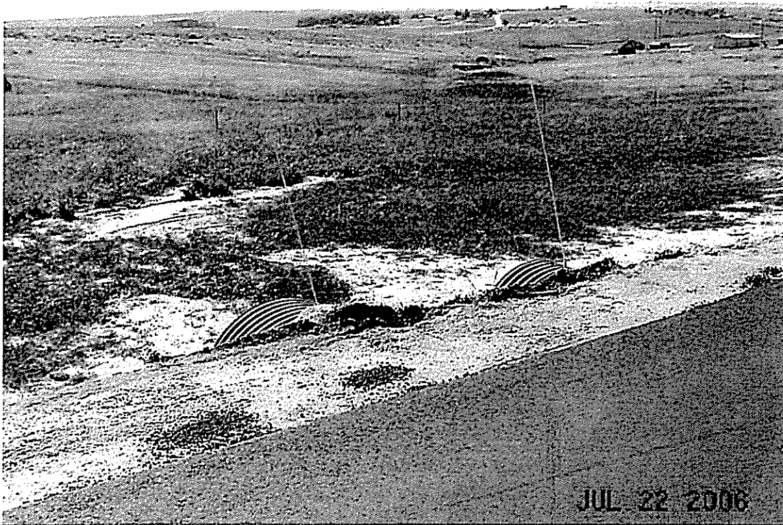
Meridian Road, Two 52" w x 34" h CMPs Outlet channel in Good Condition.
