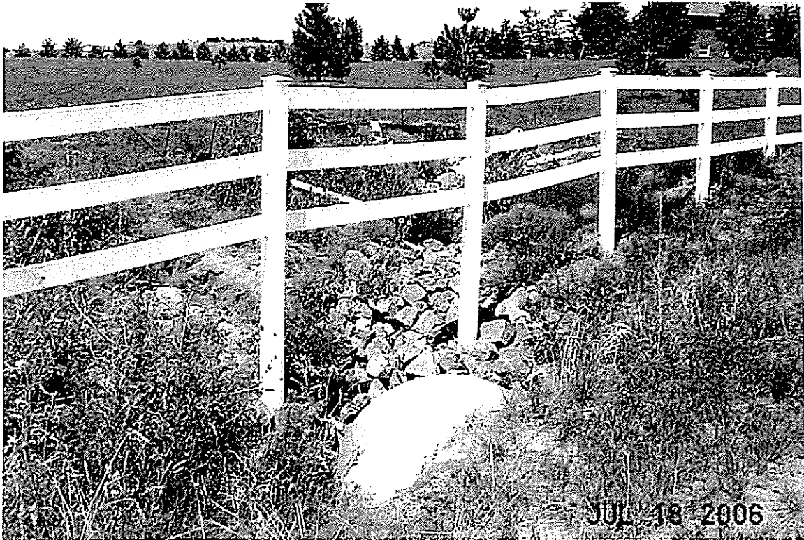
Dodge Circle, 54" w x 38" h CMP Inlet Channel in Good Condition.
