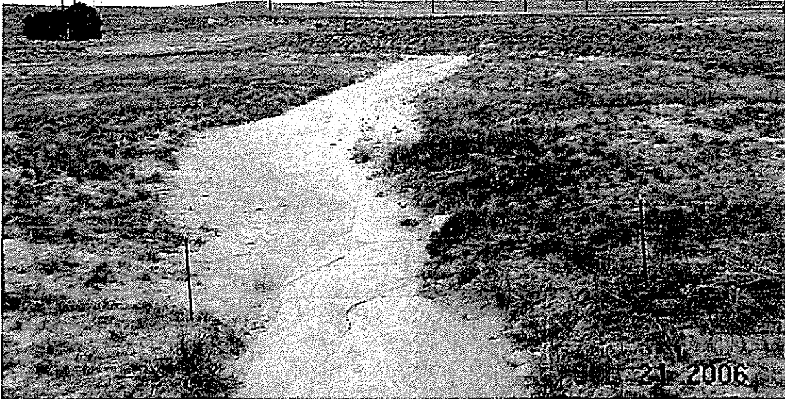
State Hwy 94, Two 8'w x 6'h Concrete Boxes Outlet Channel in Fair Condition.
