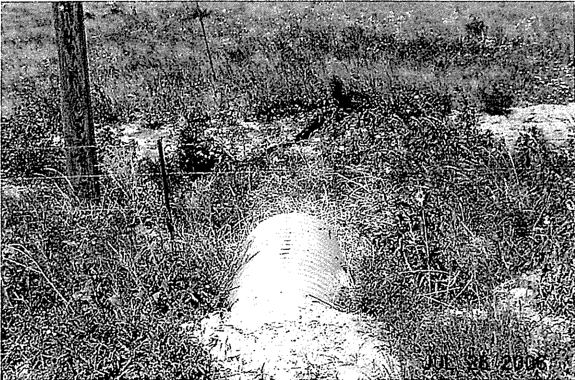
Franceville Coal Mine Road, 30" CMP Outlet Channel in Fair Condition.
