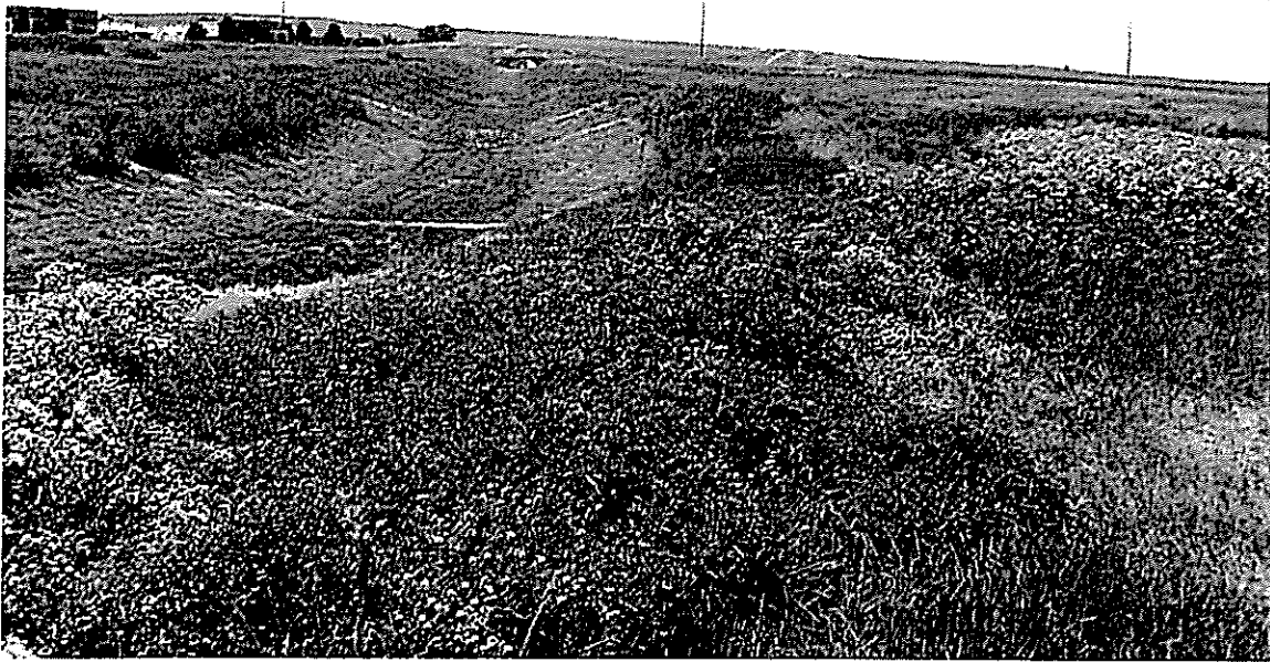
Bradley Road, 40'w Concrete Bridge Inlet Channel in Good Condition.
