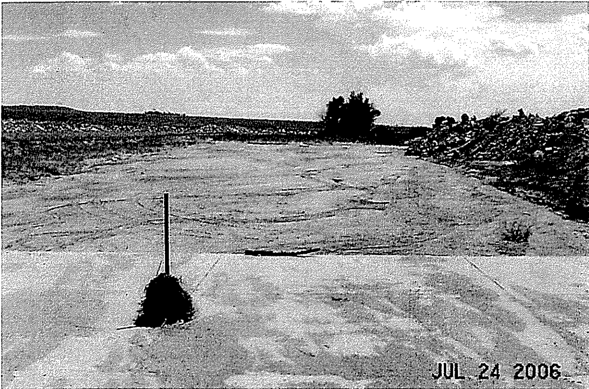
State Hwy 94, 25'w x 10'h Concrete Bridge Outlet Channel in Fair Condition.
