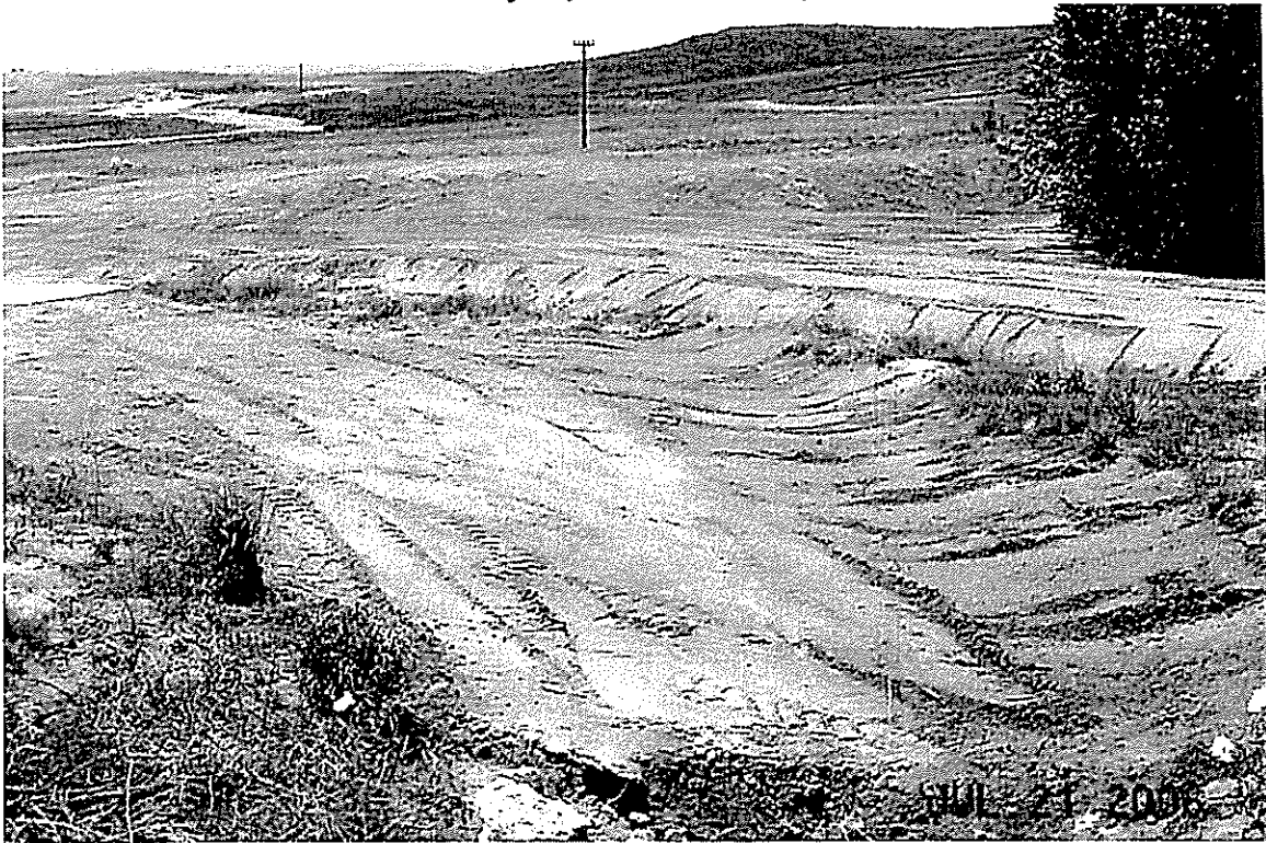
State Hwy 94, 36" CMP, Outlet Channel in Fair Condition. Appears to be drainage.
