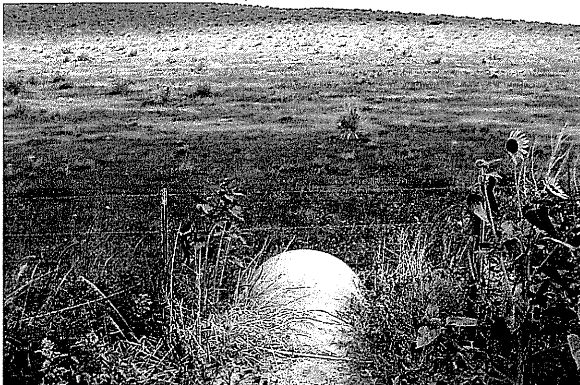
Franceville Coal Mine Road, 36" CMP Inlet Channel in Good to Fair Condition.
