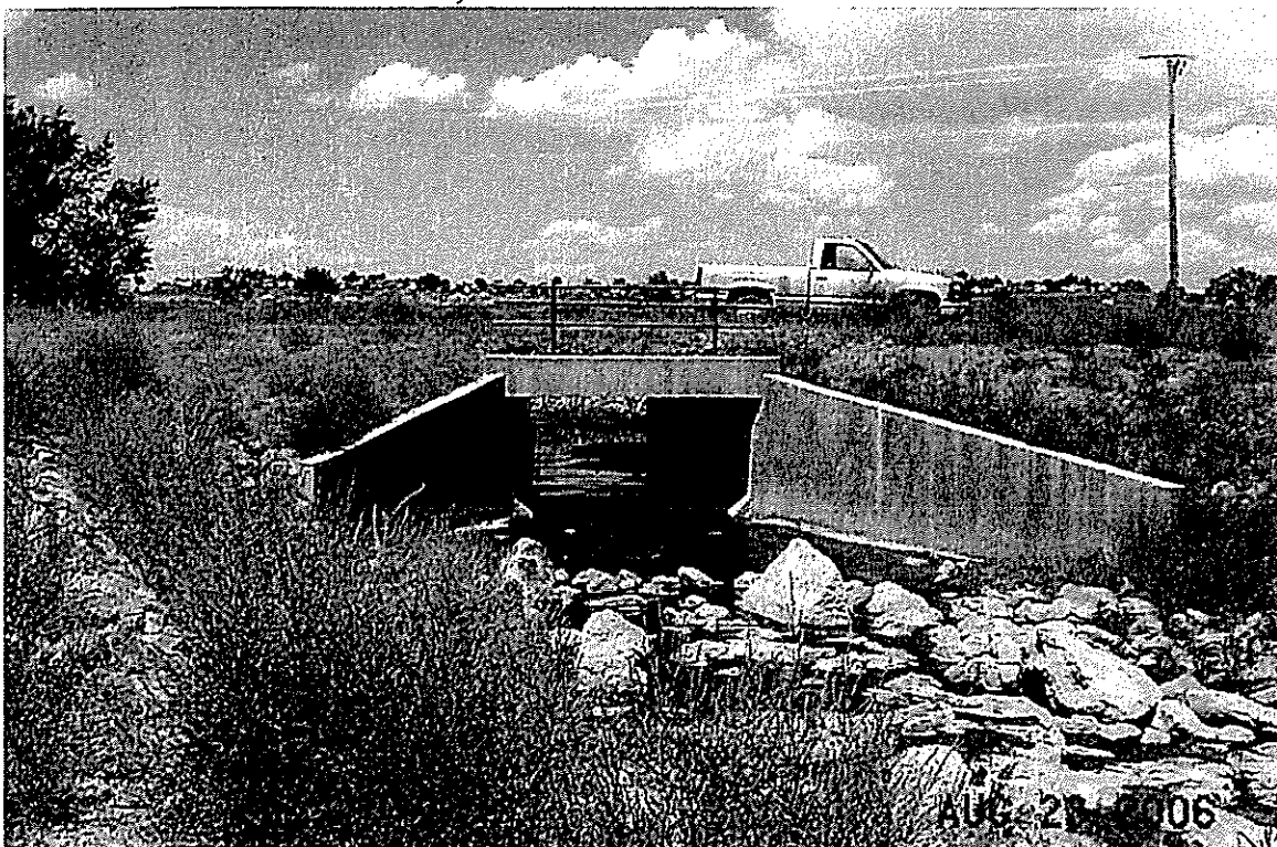
C & S Road, 12'w x 6'h concrete box culvert outlet.
