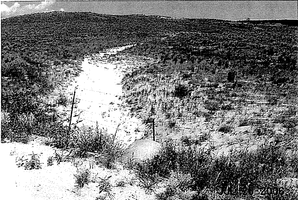
Franceville Coal Mine Road, Two 42" CMPs Inlet Channel in Fair Condition.
