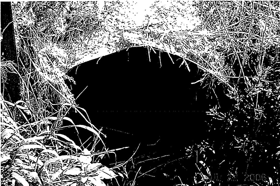
Sand Place, 30" CMP Inlet, bent.
