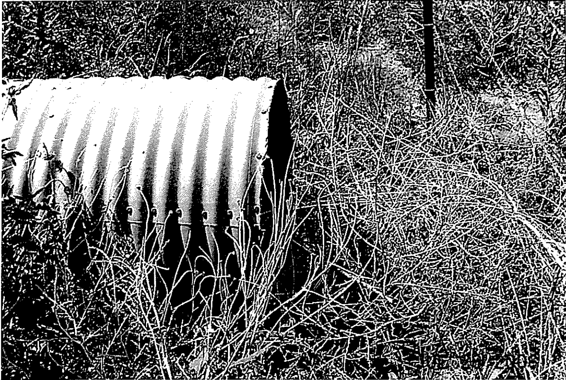
Franceville Coal Mine Road, 30" CMP Outlet.
