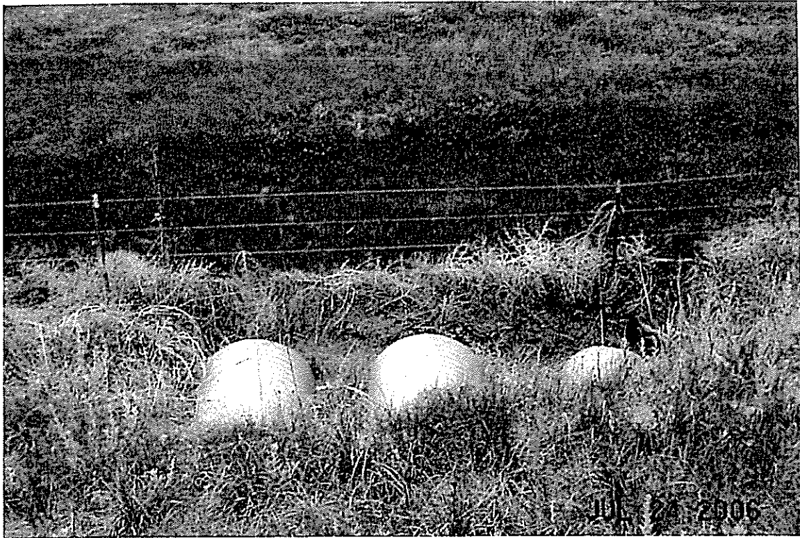
State Hwy 94, Two 36" & One 30" CMPs Inlet Channel in Fair to Good Condition.
