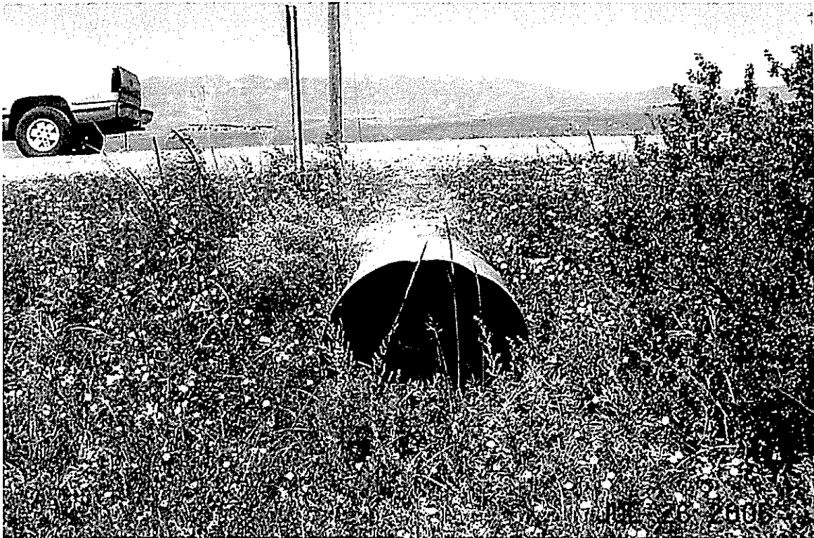
Franceville Coal Mine Road, 30" CMP Inlet.
