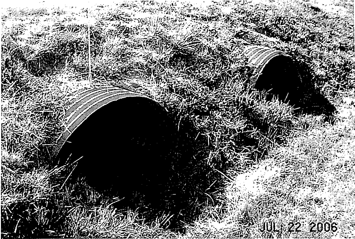
Meridian Road, Two 52" w x 34" h CMPs Inlet, bent.
