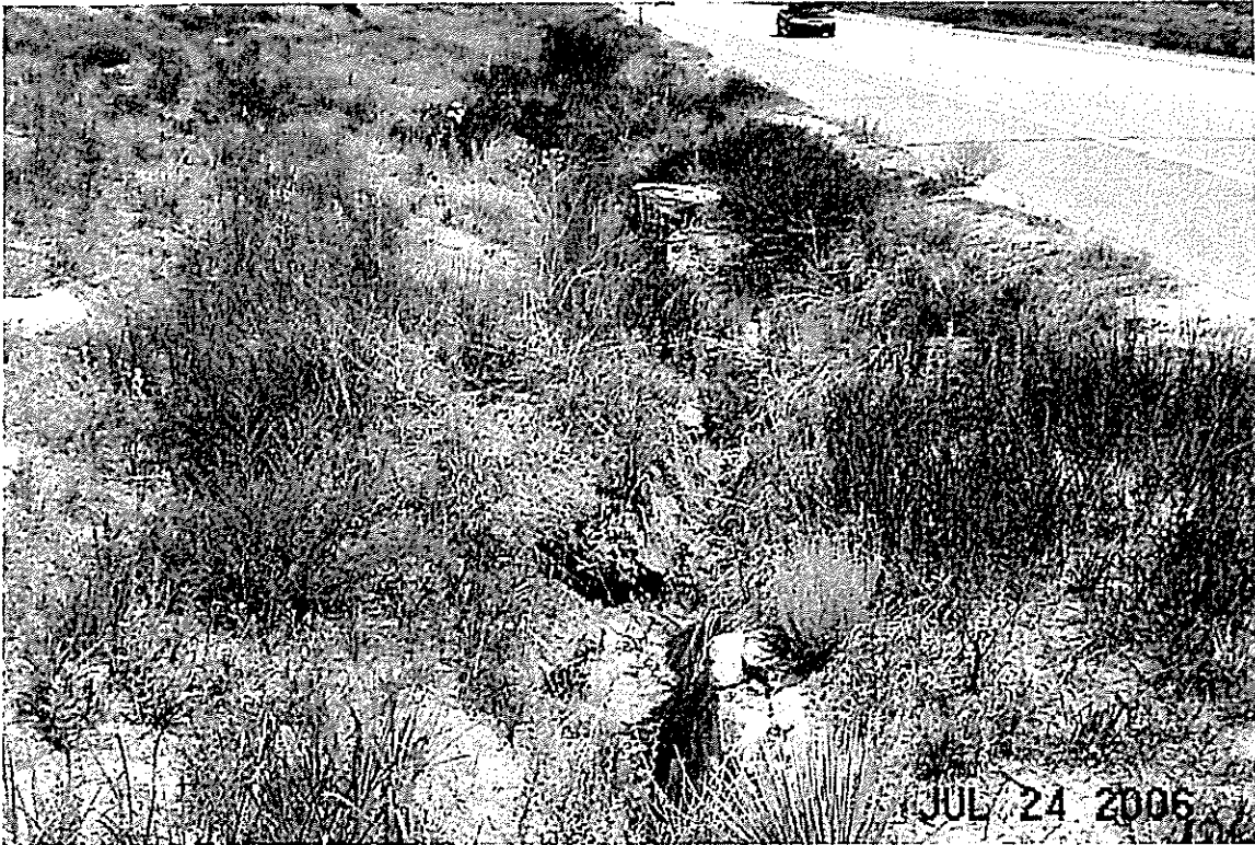
State Hwy 94, 18" CMP Inlet Channel in Fair Condition.
