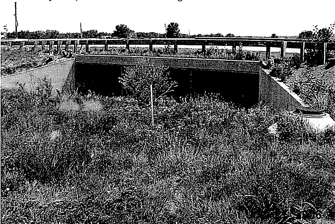
Bradley Road, 40'w x 7' h Concrete Bridge Inlet. 6
