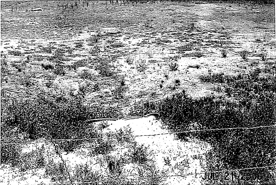
State Hwy 94, 24" CMP Outlet Channel in Fair Condition.
