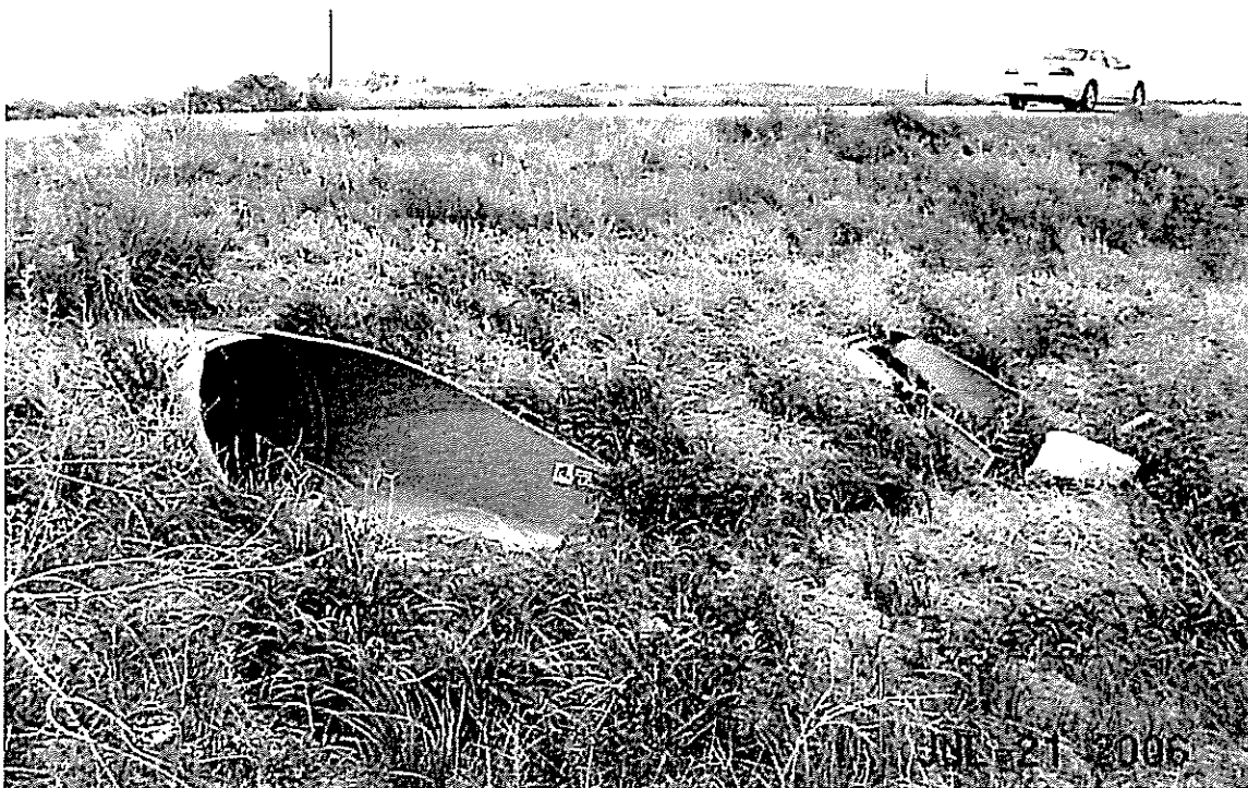
State Hwy 94, One 24" CMP & One 30" CMP Inlet in OK Condition.
