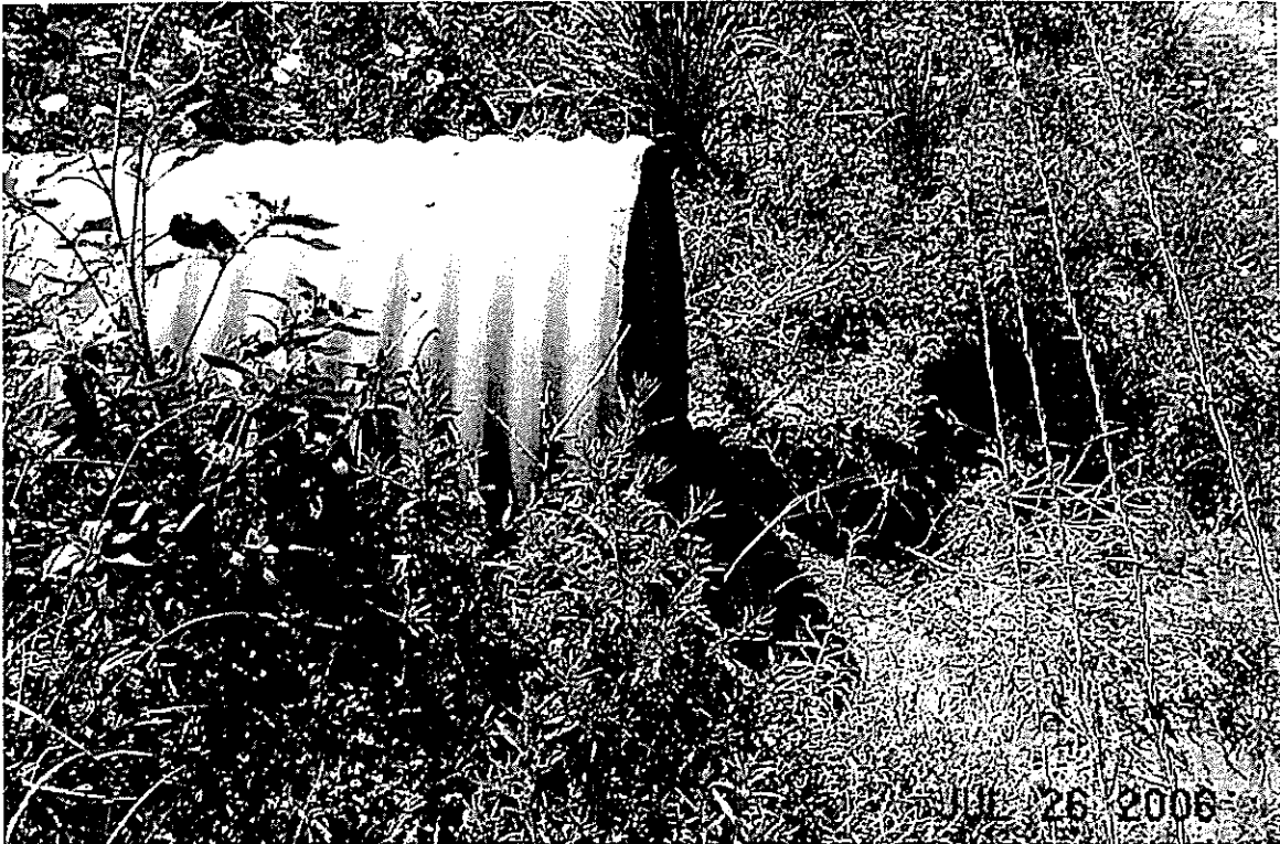
Franceville Coal Mine Road, 30" CMP Outlet.
