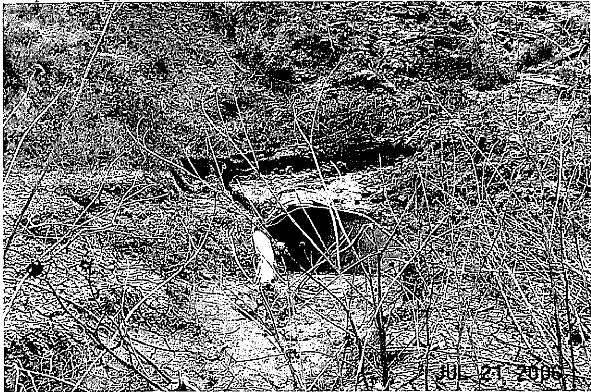
Space Village, 28" CMP Inlet, bent.
