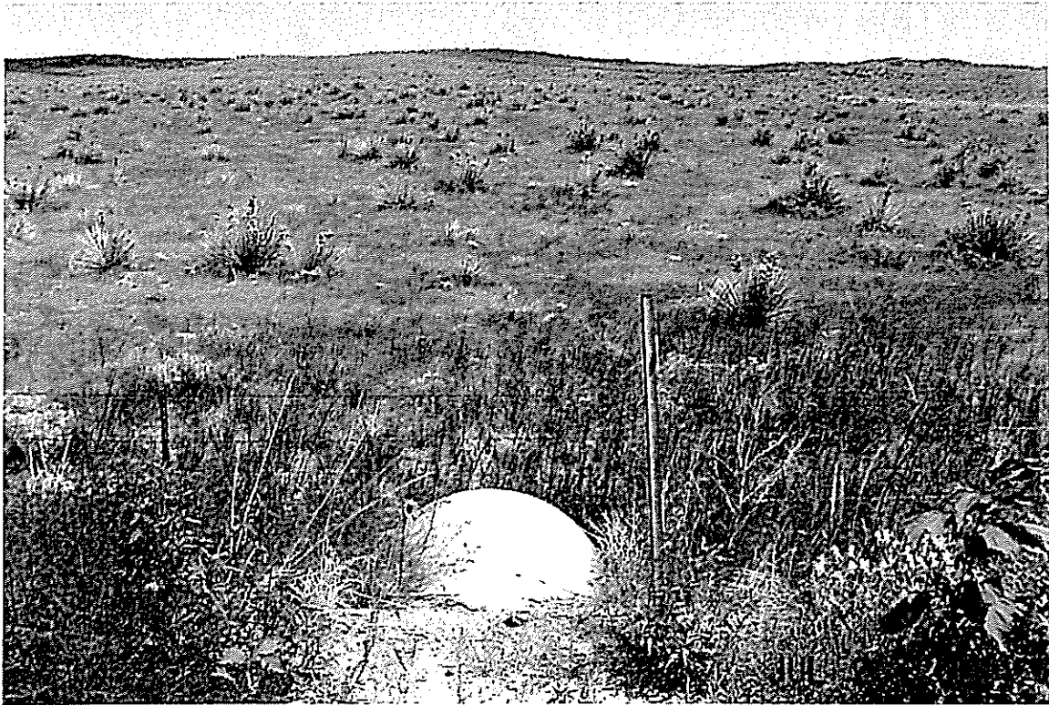
Franceville Coal Mine Road, 42" CMP Inlet Channel in Good to Fair Condition.
