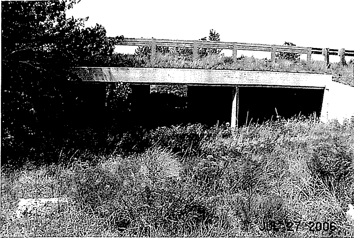
Bradley Road, 40'w x 7' h Concrete Bridge Outlet.
