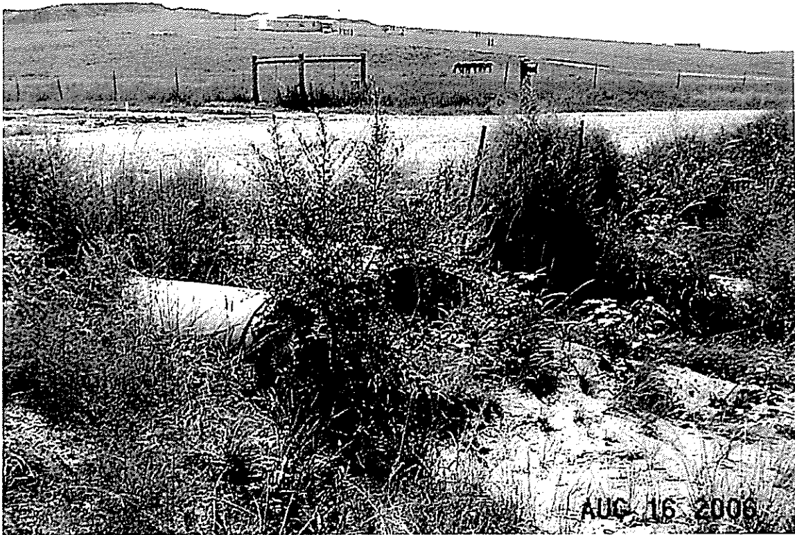
Meridian Road, two 43" w x 27" h CMPs and two 30" RCPS inlet.
