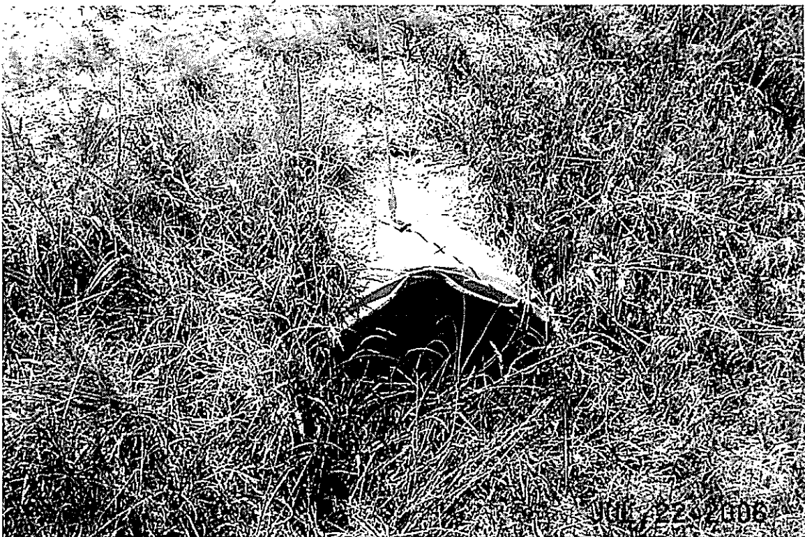
Meridian Road, 21" CMP Inlet, bent.
