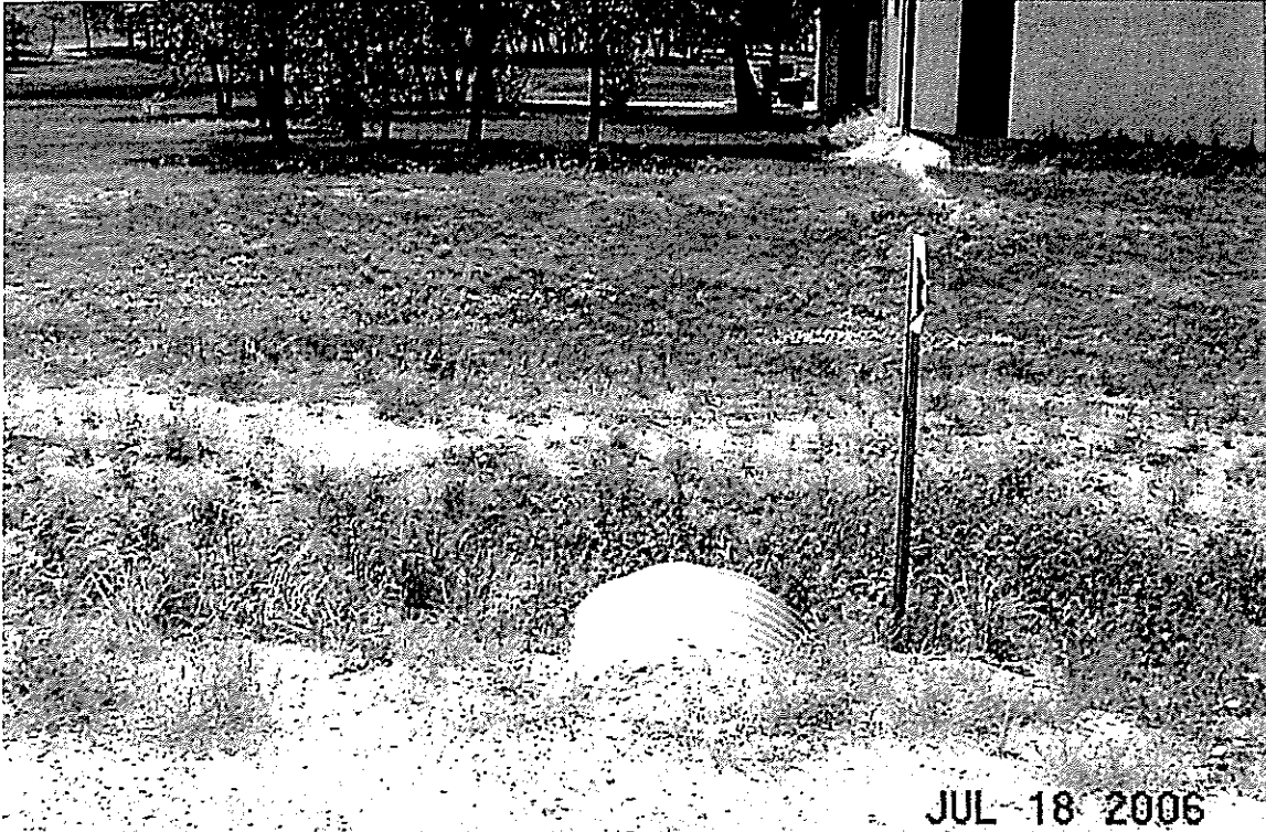
Dodge Circle, 36" CMP Inlet Channel in Fair Condition.
