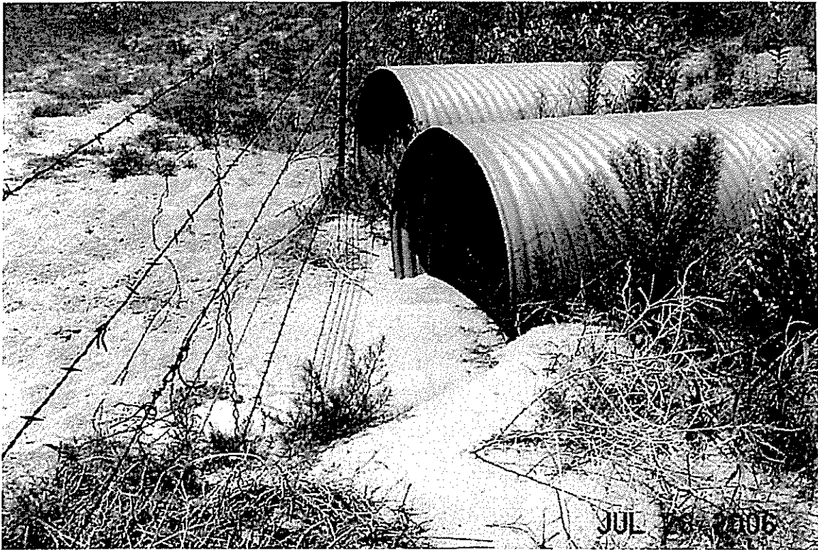
Franceville Coal Mine Road, Two 42" CMPs Outlet.
