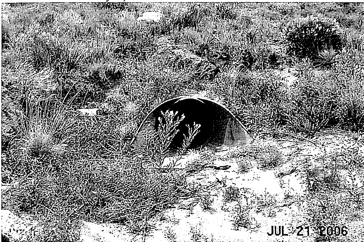
State Hwy 94, 36" CMP Inlet, bent.
