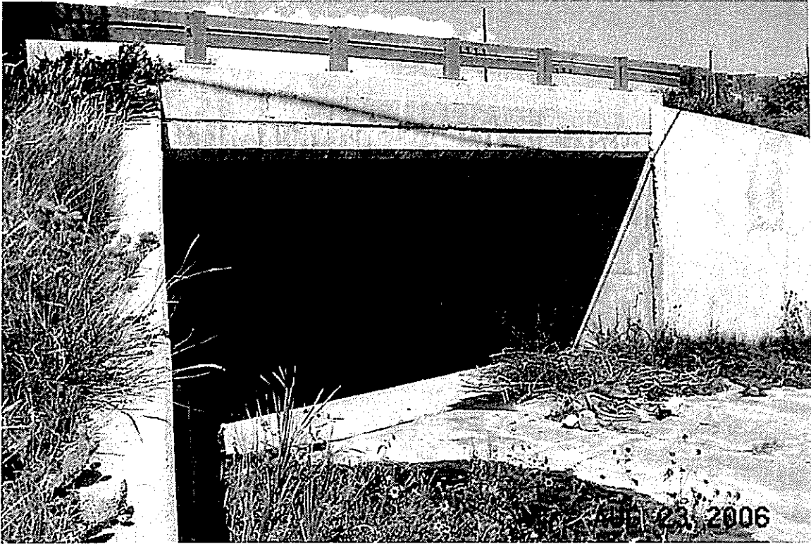
Fontaine Road, 26'w x 10'h Box Culvert outlet.
