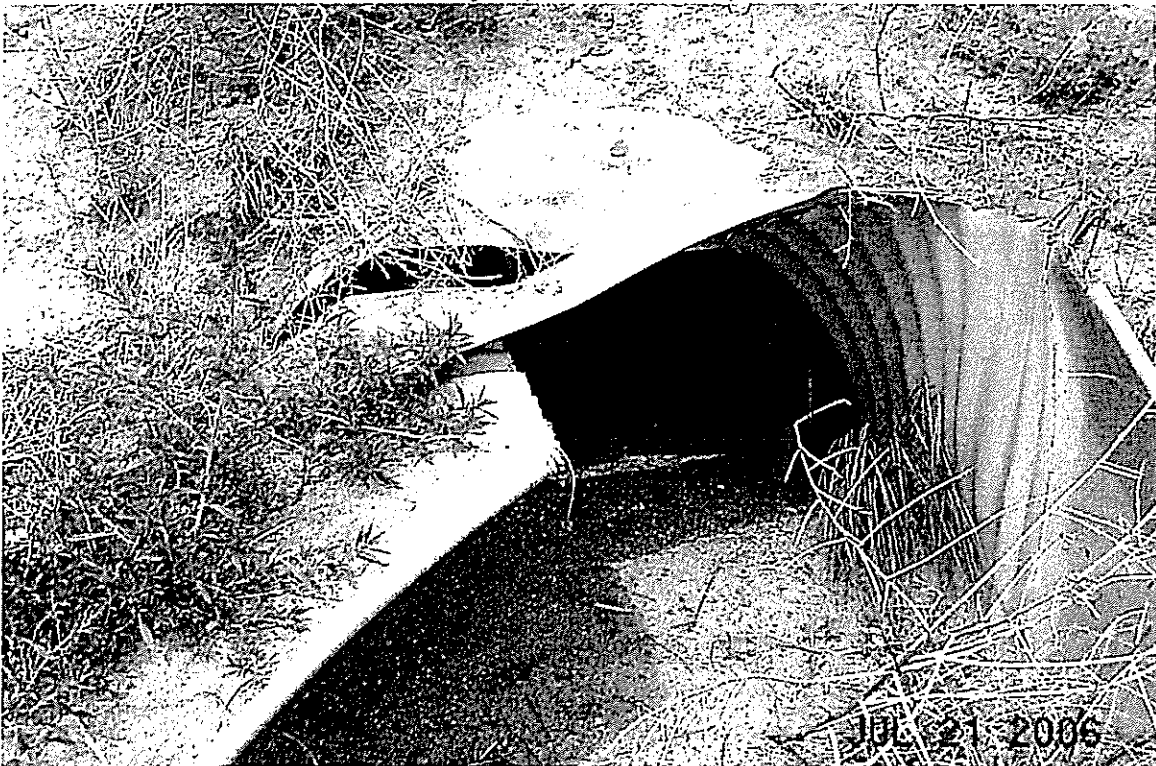
State Hwy 94, 48" CMP Outlet, bent.
