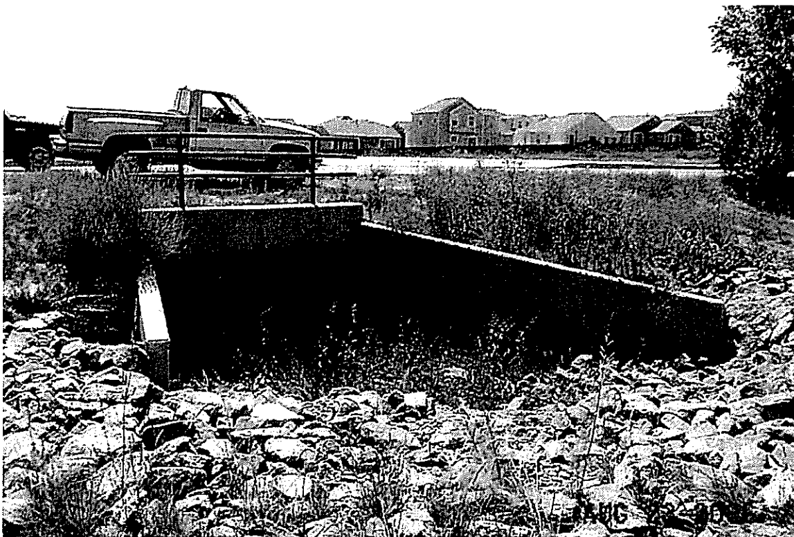
C & S Road, 12'w x 6'h concrete box culvert inlet.
