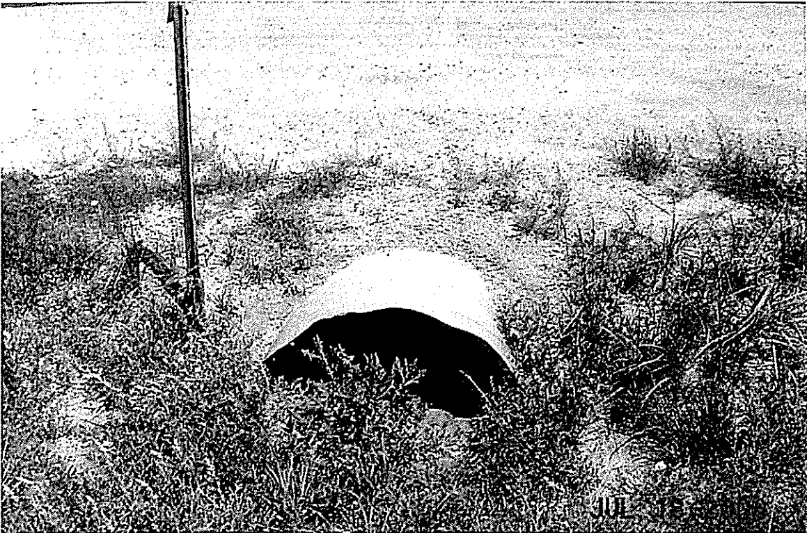
Dodge Circle, 36" CMP Inlet, bent.
