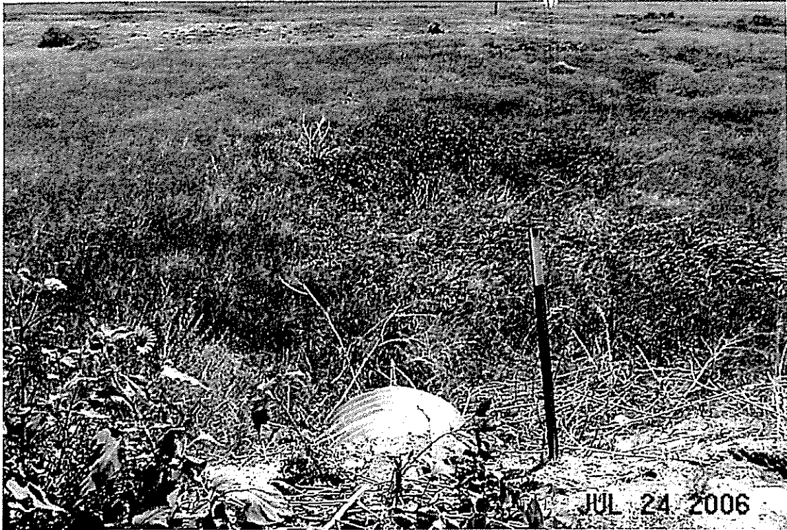
Corral Valley Road, 30" CMP Inlet Channel in Good Condition.
