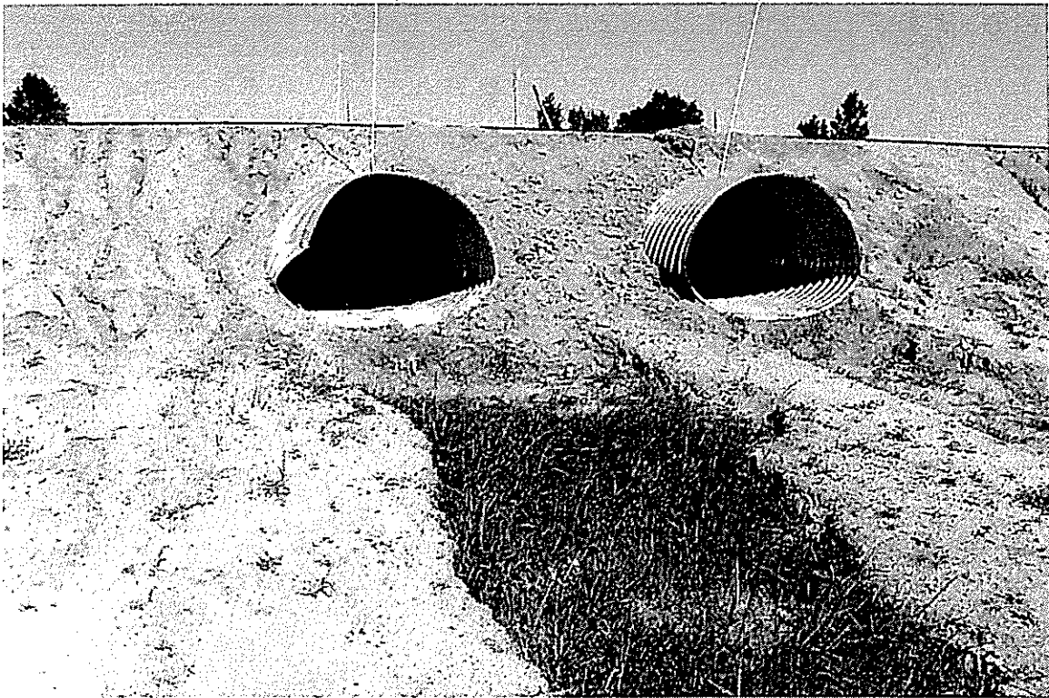
Meridian Road, Two 52" w x 34" h CMPs Outlet, bent.
