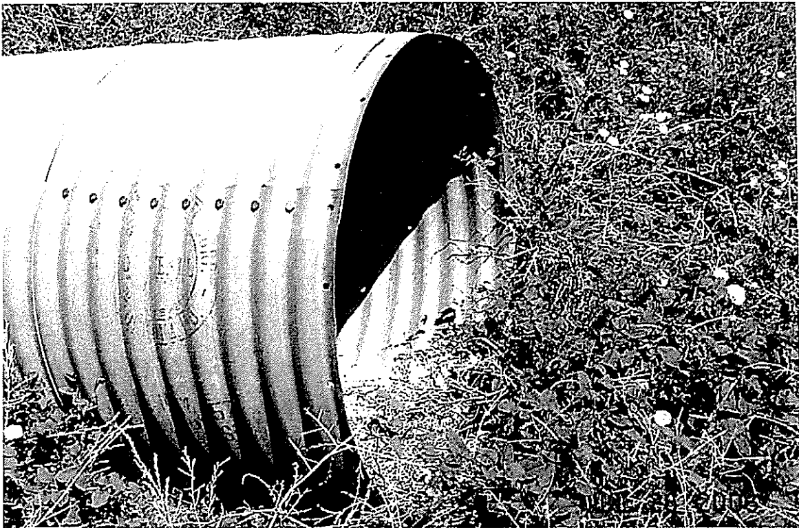
Franceville Coal Mine Road, 36" CMP Inlet.
