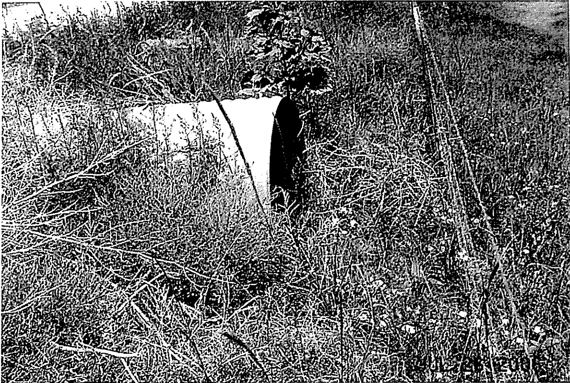
Franceville Coal Mine Road, 36" CMP Inlet.
