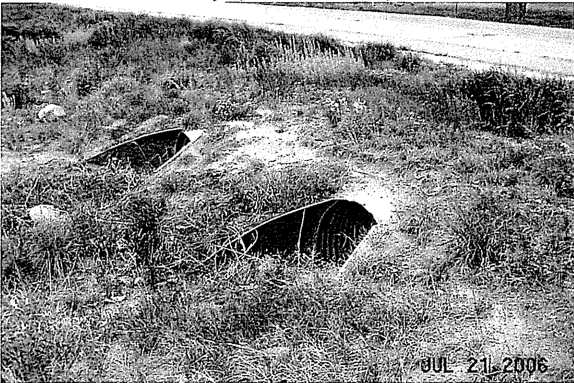
State Hwy 94, Two 48" CMPs Outlets, OK.
