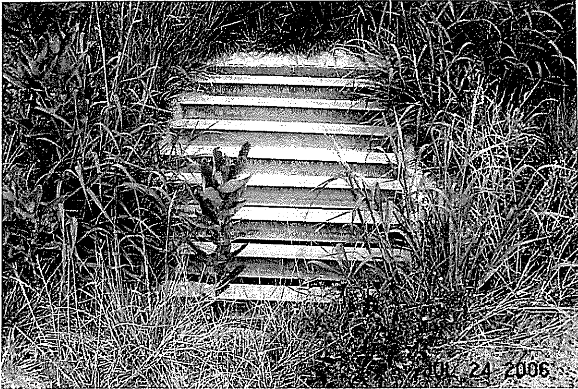
State Hwy 94, 68" x 36" Type C or D Inlet.
