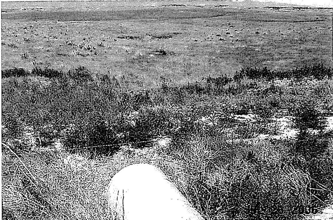
Franceville Coal Mine Road, 36" CMP Inlet Channel in Good Condition.
