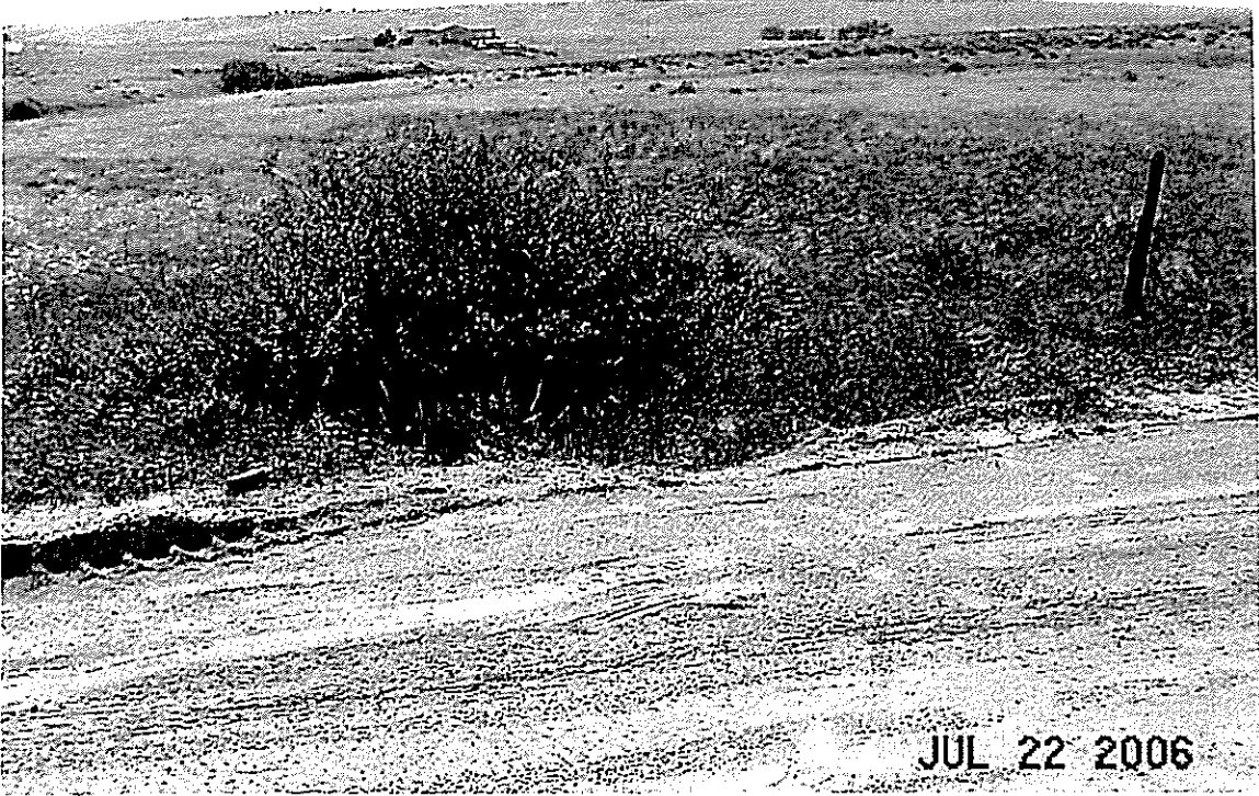
Meridian Road, 18" CMP Outlet channel in Good Condition.
