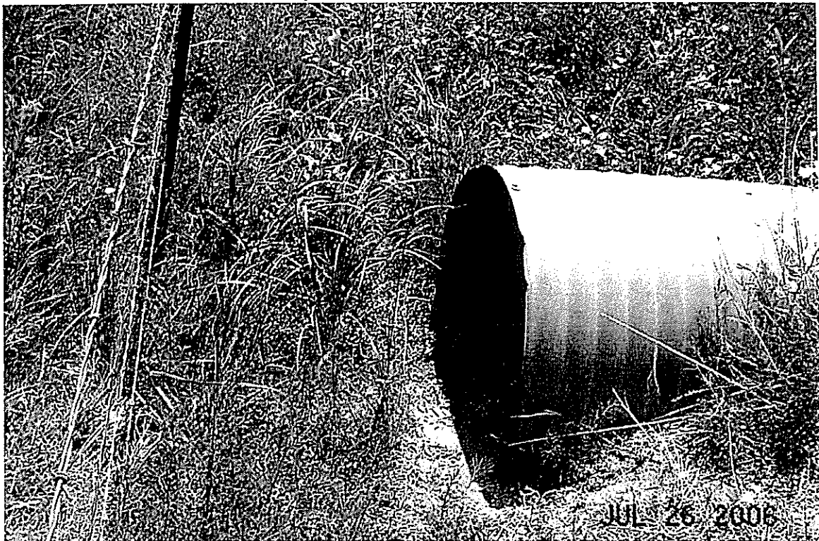
Franceville Coal Mine Road, 30" CMP Inlet.
