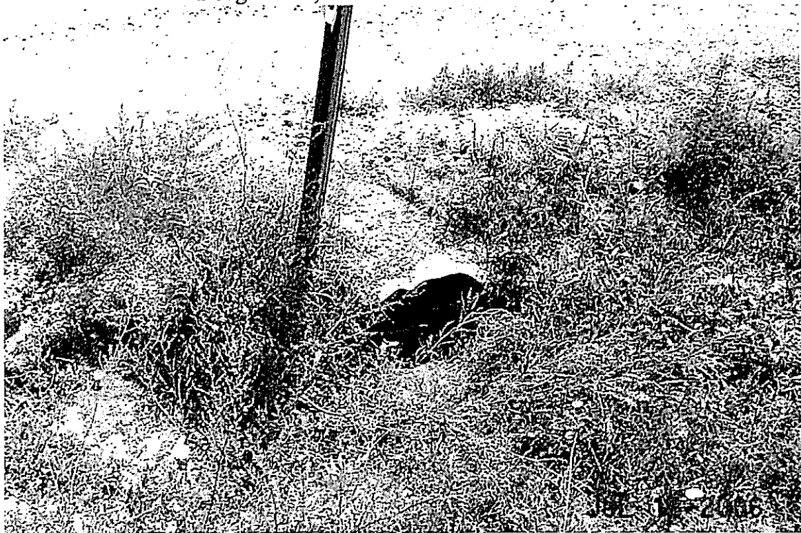
Dodge Circle, 21" CMP Inlet, bent. Inlet Channel Fair.
