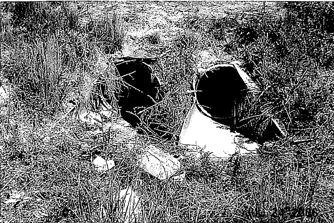
State Hwy 94, Two 24" CMPs Inlet, bent.
