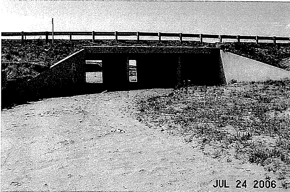
State Hwy 94, 37'3"w x 10'h Concrete Bridge Inlet.
