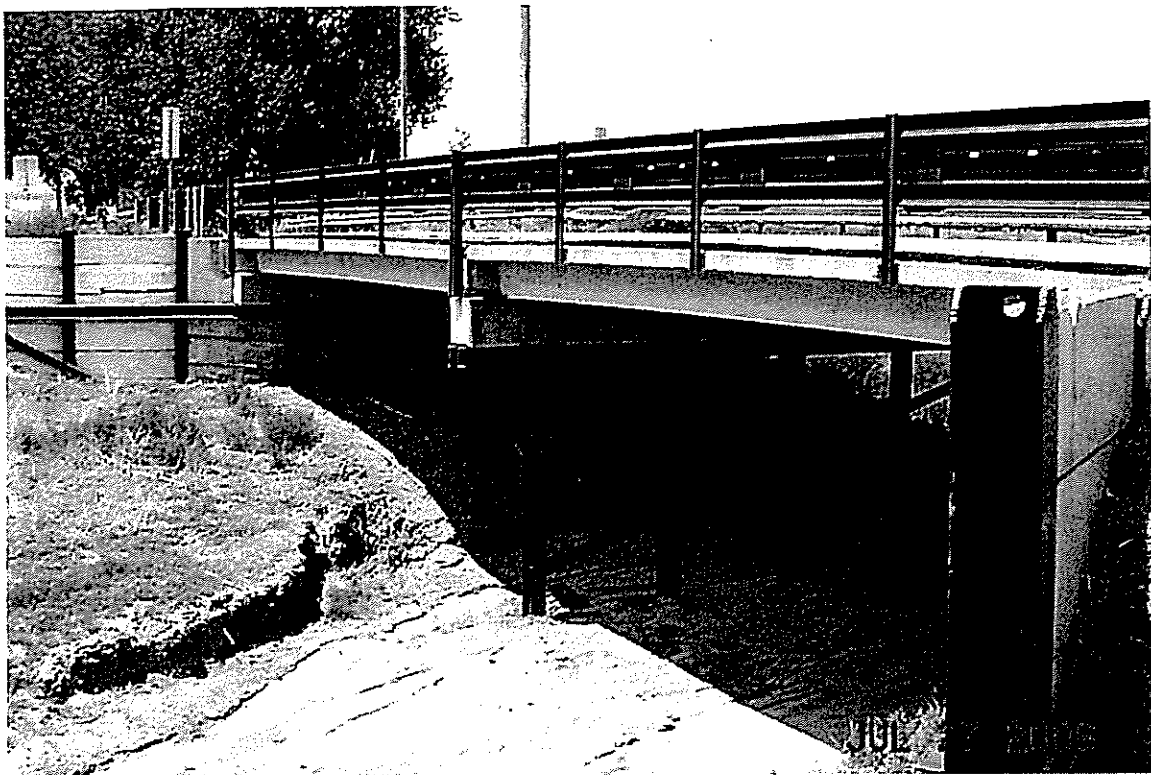
Drennan Road, 54'w x 12'h Concrete and Steel Bridge Outlet.
