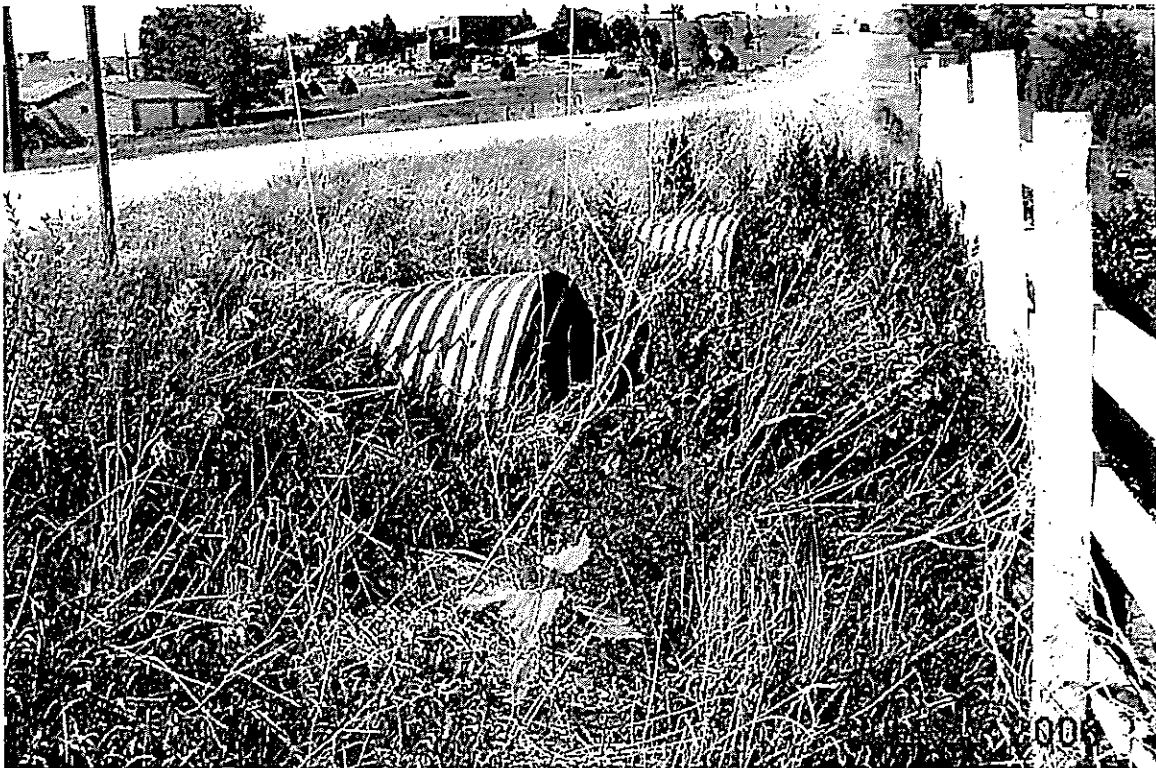
Meridian Road, Two 58" w x 36" h CMPs Inlet, bent.
