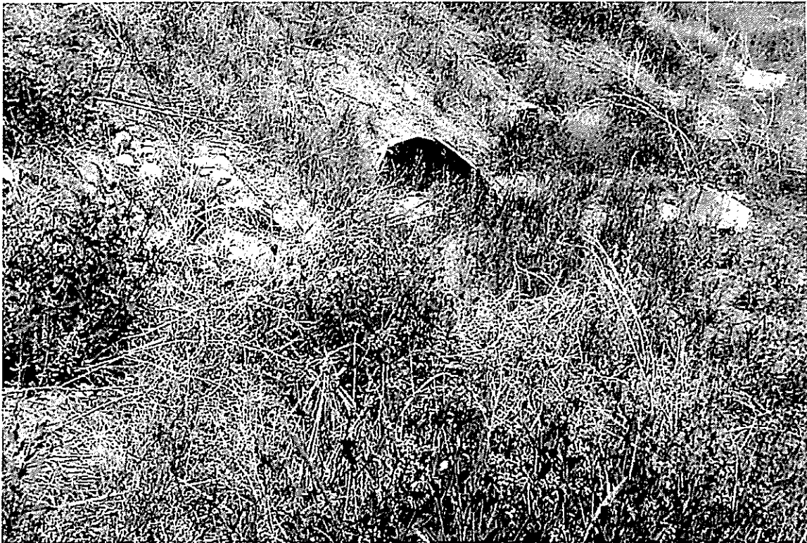
State Hwy 94, Three 36" CMPs Outlet, bent.
