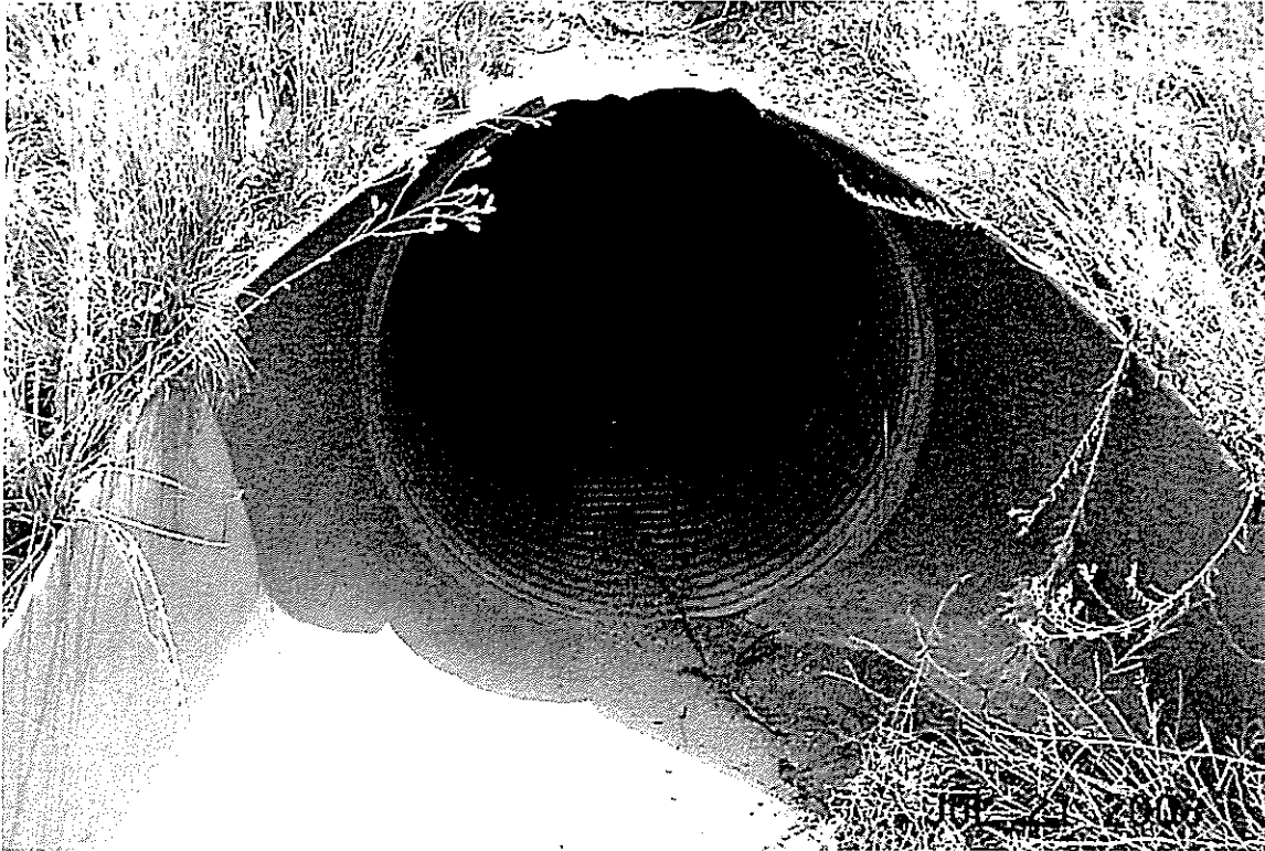
State Hwy 94, 48" CMP Inlet, bent.
