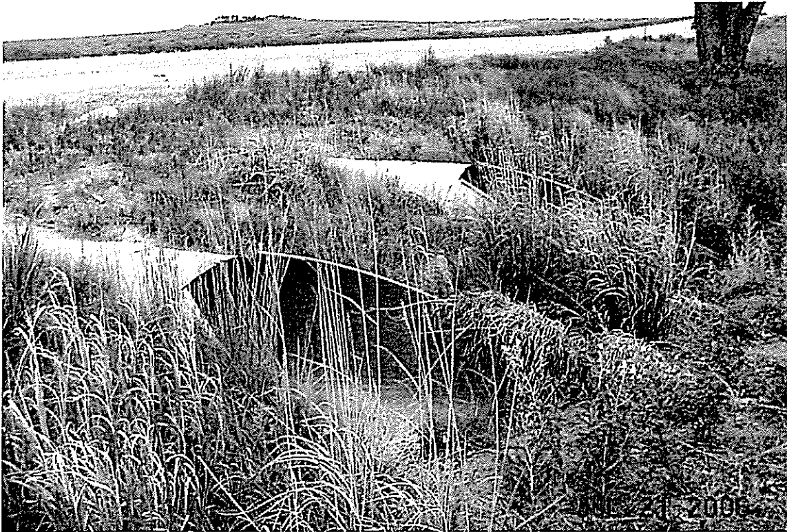
State Hwy 94, Two 48" CMPs Inlets, OK.
