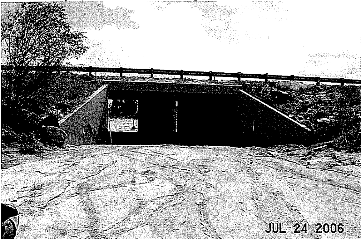
State Hwy 94, 25'w x 10'h Concrete Bridge Inlet.
