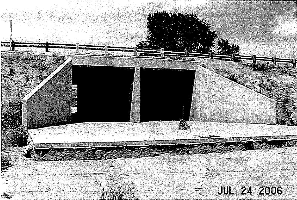
State Hwy 94, 25'w x 10'h Concrete Bridge Outlet.
