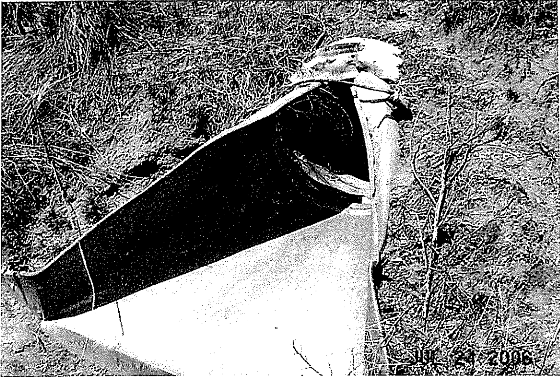
State Hwy 94, 24" CMP Outlet, bent.
