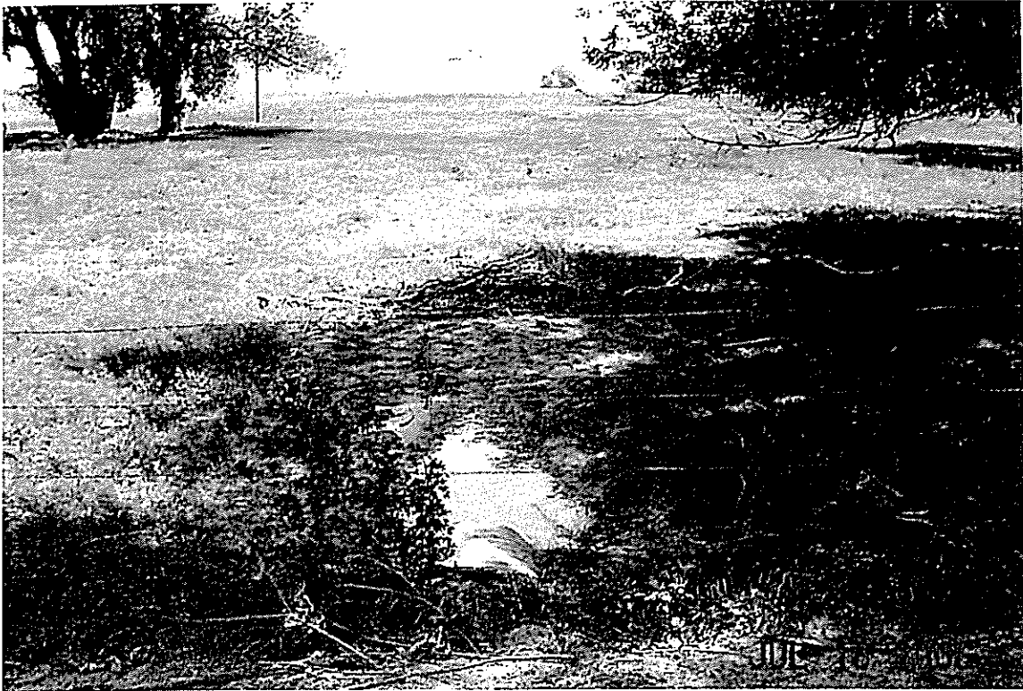
Dodge Circle, 24" CMP Outlet Channel, Outlet Channel Fair. Appears to be drainage.
