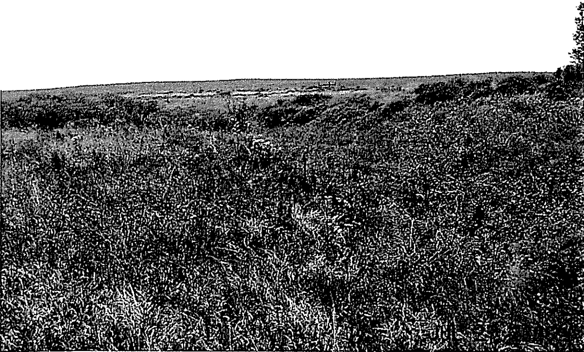
Bradley Road, 40'w x 7' h Concrete Bridge Outlet Channel in Good Condition.
