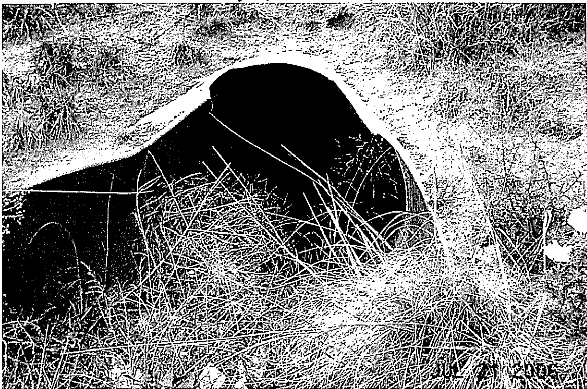
State Hwy 94, 48" CMP Outlet, bent.
