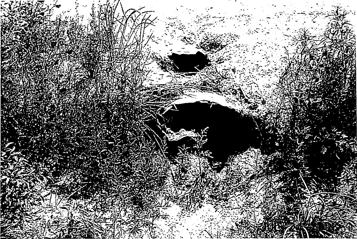
Corral Valley Road, 24" CMP Outlet, bent and damaged.
