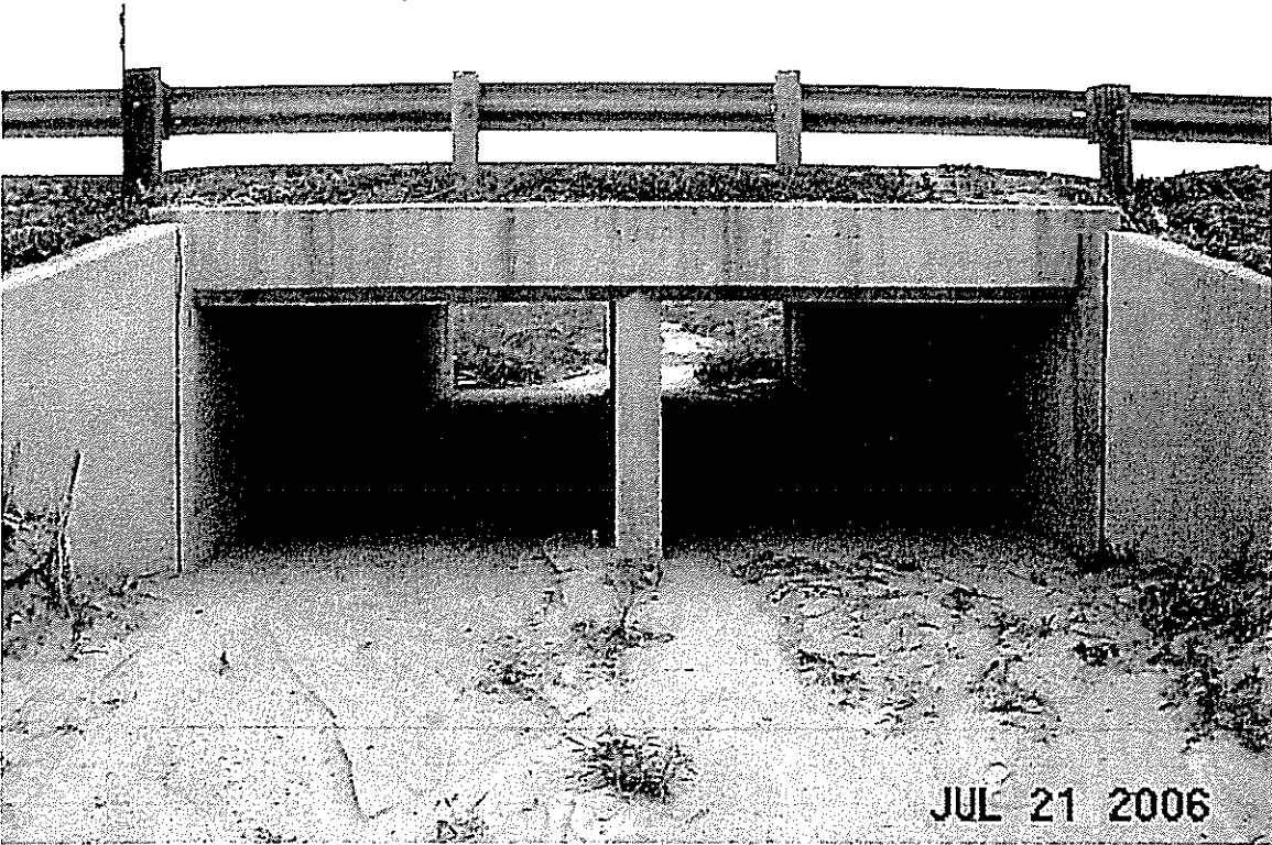
State Hwy 94, Two 8'w x 6'h Concrete Boxes Outlet.
