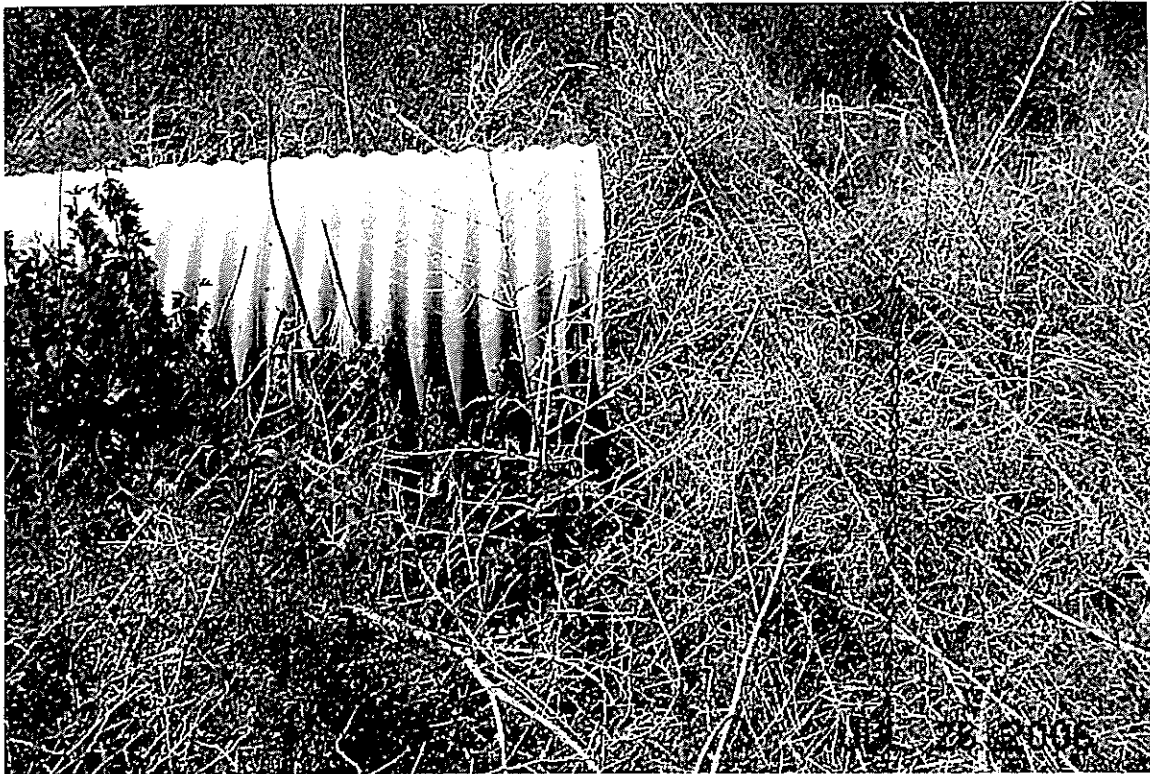
Franceville Coal Mine Road, 36" CMP Outlet.
