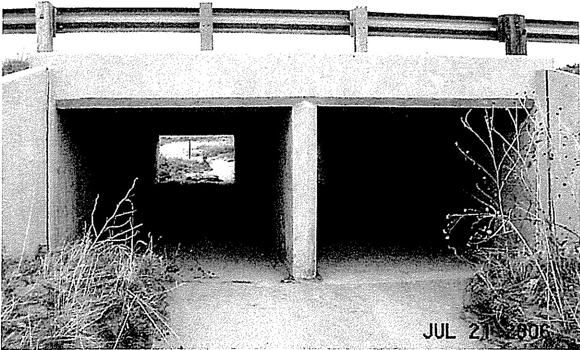
State Hwy 94, Two 8'w x 6'h Concrete Boxes Inlet.
