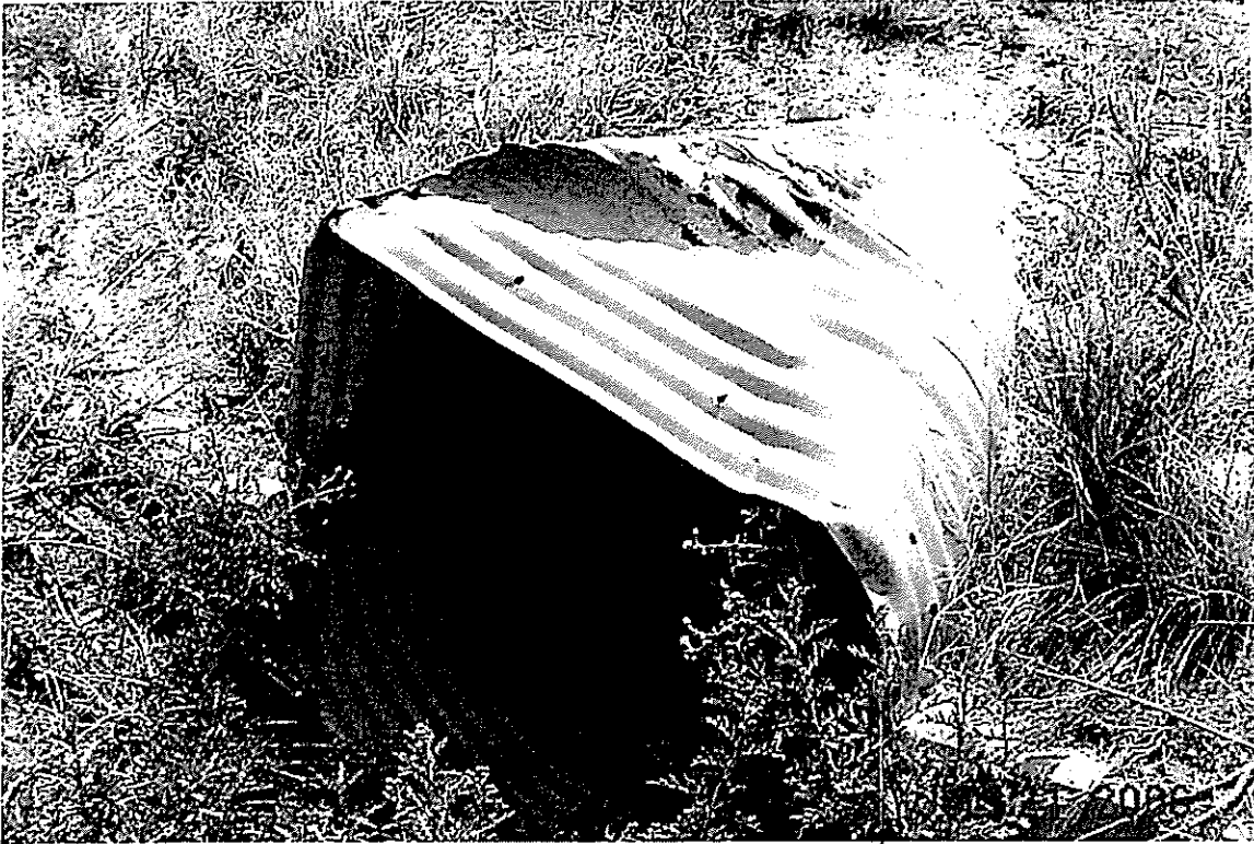
State Hwy 94, 54" CMP Inlet, bent.
