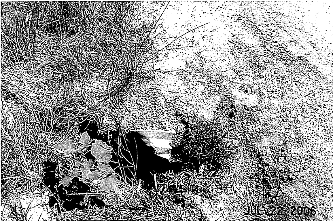
Smith Road, 21" CMP Inlet, Bent.
