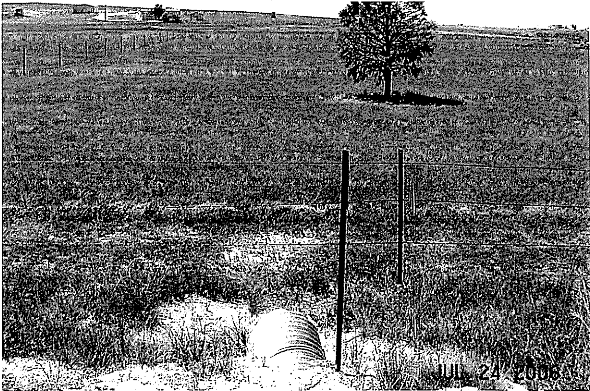
West Lane, 18" CMP Outlet Channel in Fair to Good Condition.
