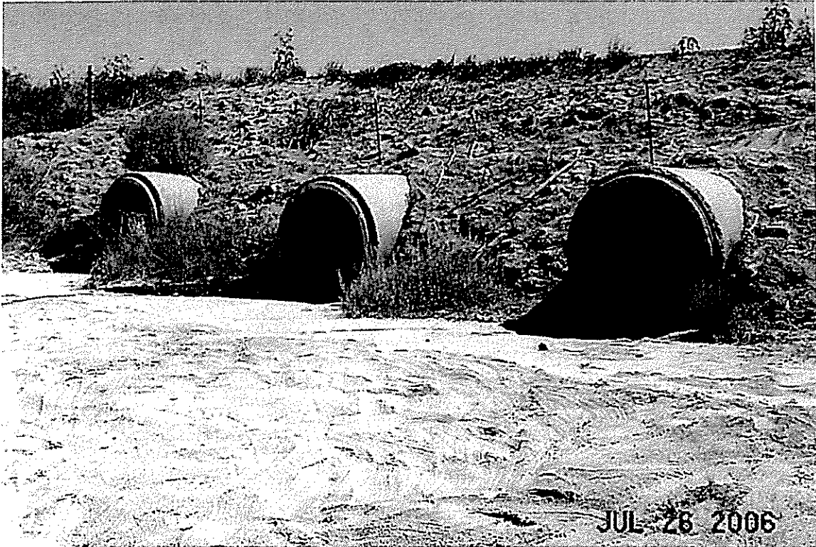
Franceville Coal Mine Road, Three 60" RCPs Outlet.
