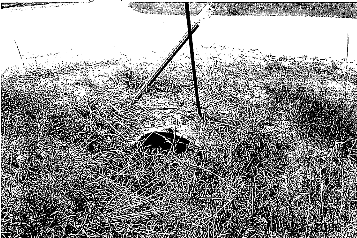
Partridge Lane, 30" CMP Inlet, bent.
