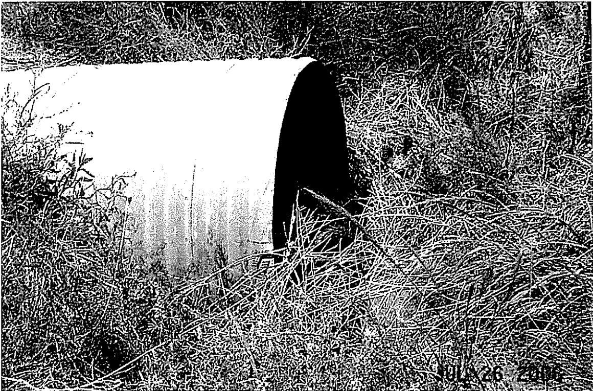
Franceville Coal Mine Road, 42" CMP Inlet.
