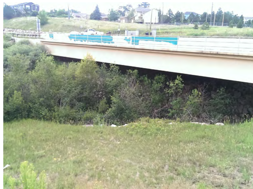
OLD RANCH ROAD BRIDGE LOOKING NORTH
