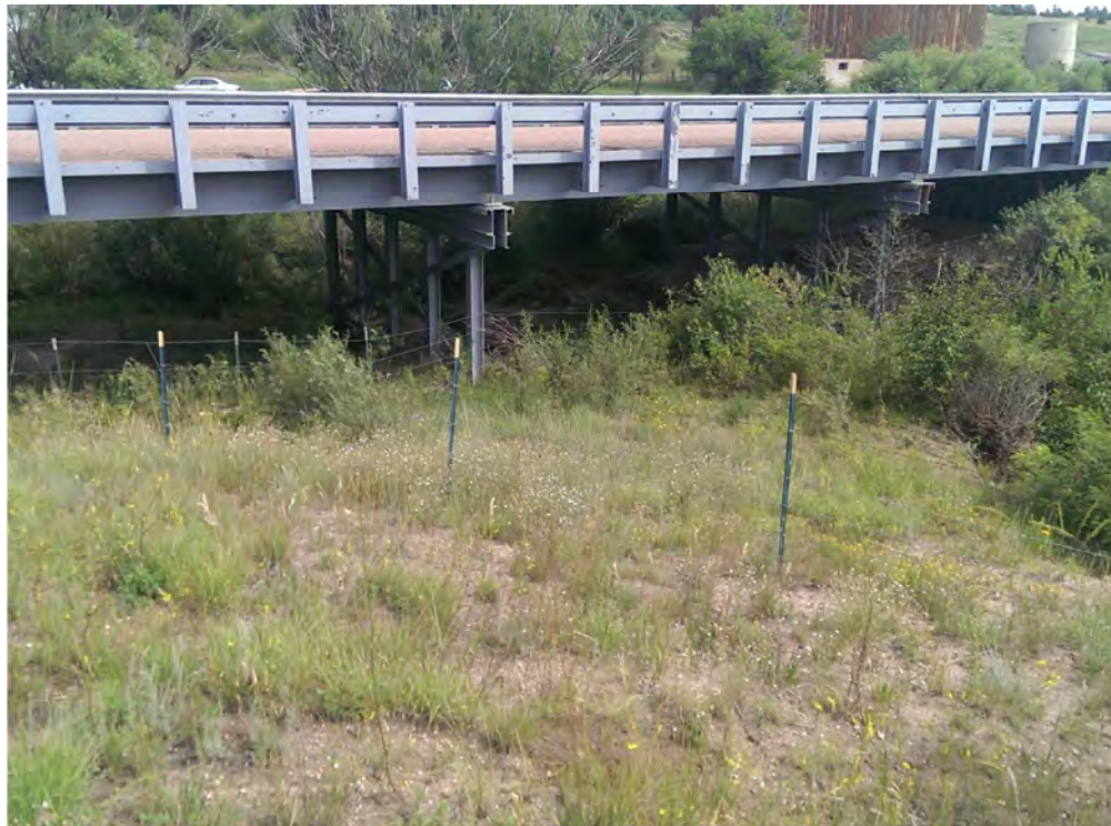
OTERO AVE BRIDGE LOOKING UPSTREAM
