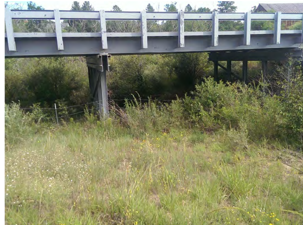
OTERO AVE BRIDGE LOOKING UPSTREAM
