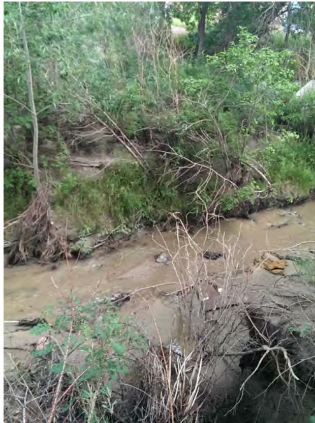
CHANNEL CONDITIONS APPROX. STA 169+00
