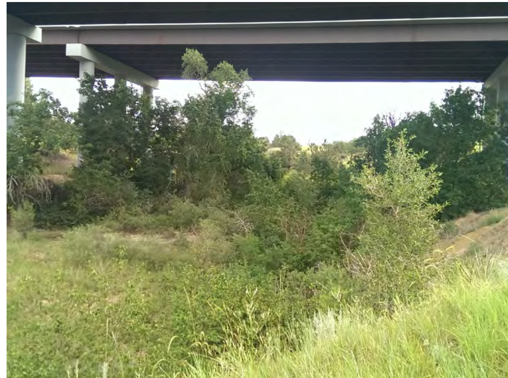
POWERS BLVD BRIDGE LOOKING UPSTREAM
