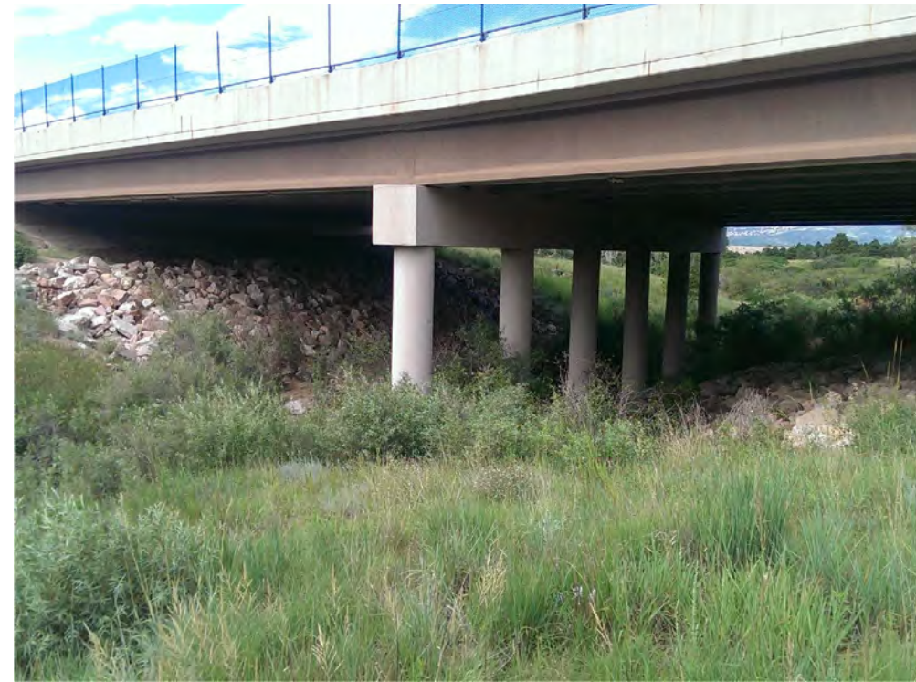
HWY 83 BRIDGE LOOKING UPSTREAM
