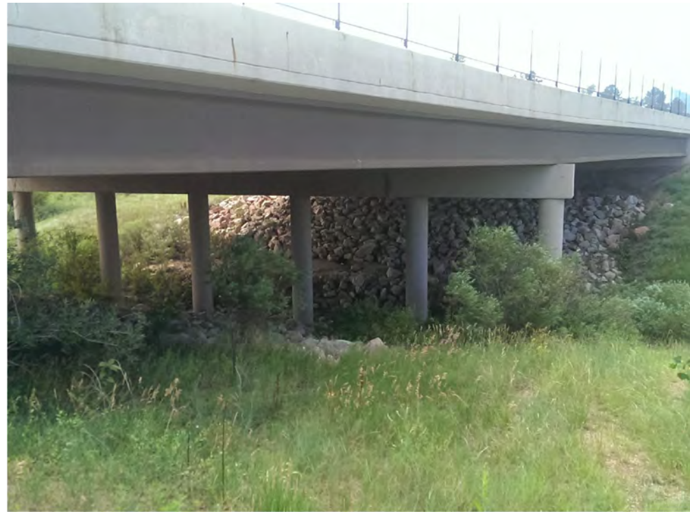
HWY 83 BRIDGE LOOKING NORTH
