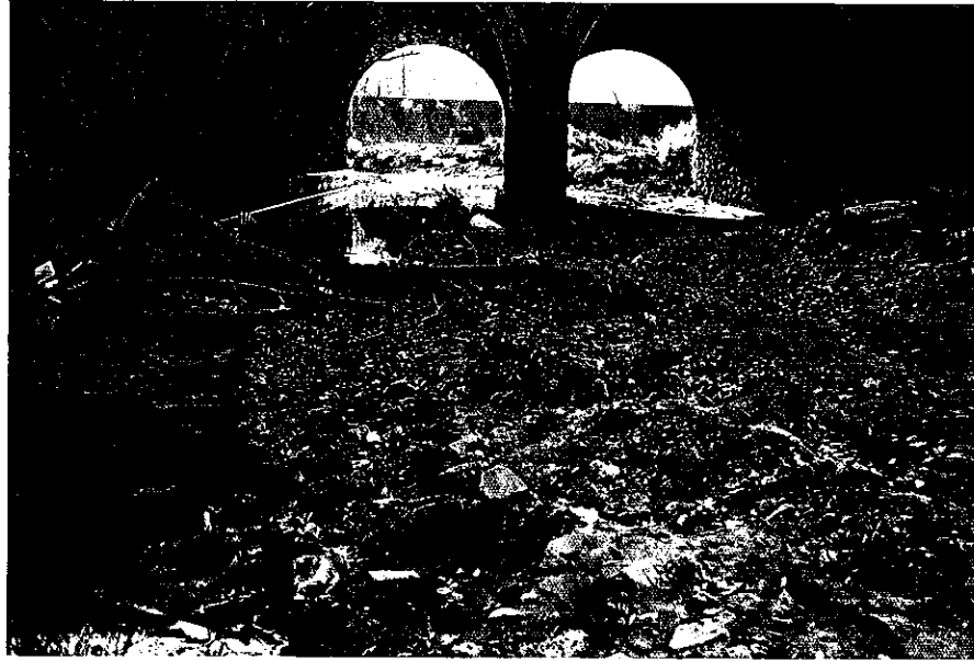
No. 15 Shown here are the large railroad arches downstream from Fountain Boulevard: Note debris and trash that collects in the channel after storm flows have subsided.
