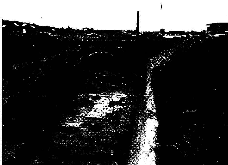
No. 2 Shown here are newly installed elliptical pipes just west of Union Boulevard. These pipes are designed to carry a peak design flow of 1646.0 CFS.
