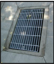
C/DOT Type C Grate (Close Mesh)
