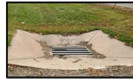
C/DOT Type C Inlet in Depression
