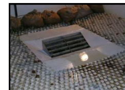
C/DOT Type D Inlet Parallel (30" Incline & Depressed)
