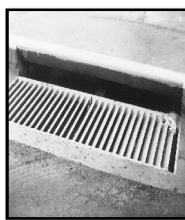
Directional 45-Degree Bar Grate
