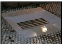
C/DOT Type D Inlet Parallel (Flat & Depressed)
