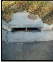
C/DOT Type A Curb Opening
