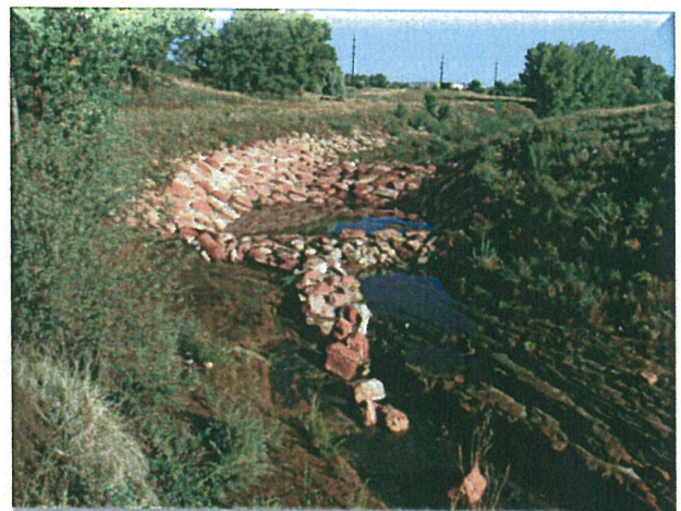
Photo 8-West Fork sewer crossing 2011
