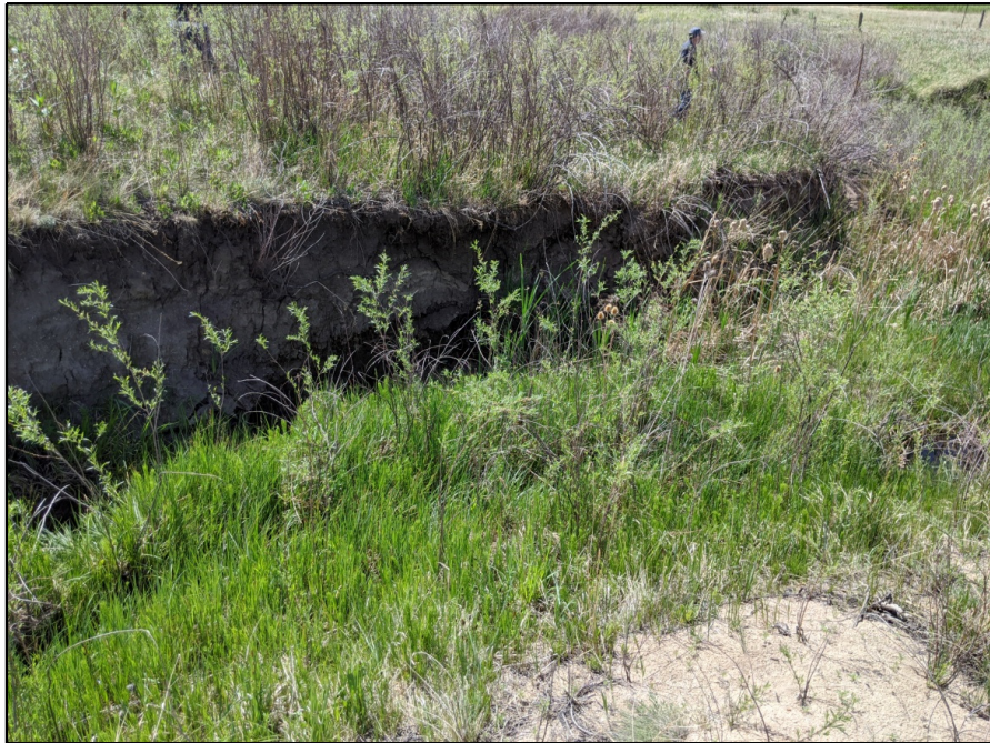
Photo 1: Looking north near XS 104
