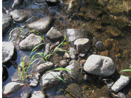
Photograph 8-18. Void-filled riprap is designed to emulate natural riffles, consisting of a mix of rock, gravels and sands that is densely-packed and able to support riparian vegetation.
