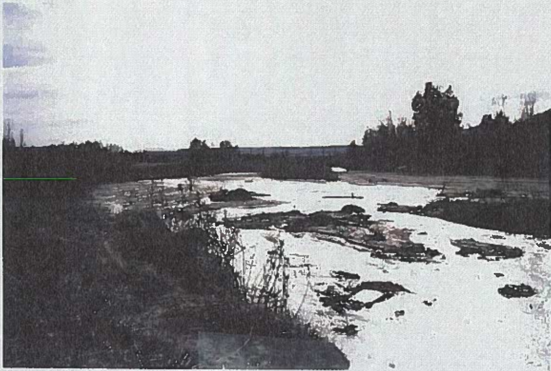
Sand Creek - 11/3/97 North of Sta. 165+00 Looking South from East Bank at Existing Pedestrian Bridge
