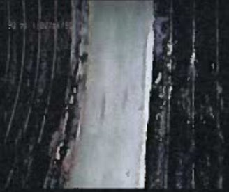
Corroded and damaged pipe is cleaned and patched.
