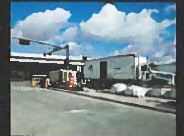
DOT projects: highways and bridge overpasses
