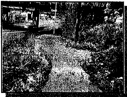
Sediment accumulation at Tejon Street and railroad intersection at 20' inlet
