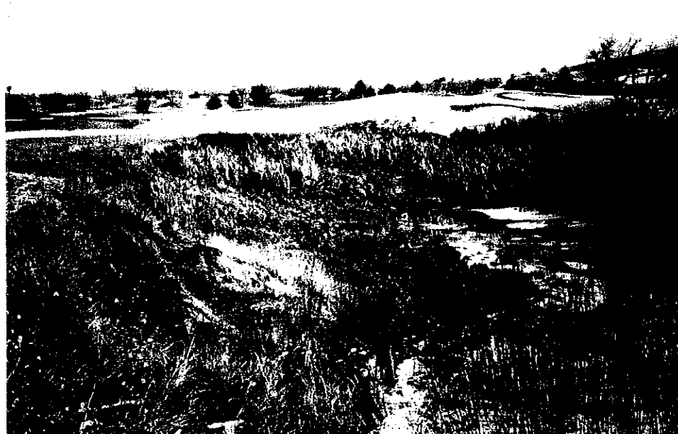
10. Unstable North Bank. MP 3.14
