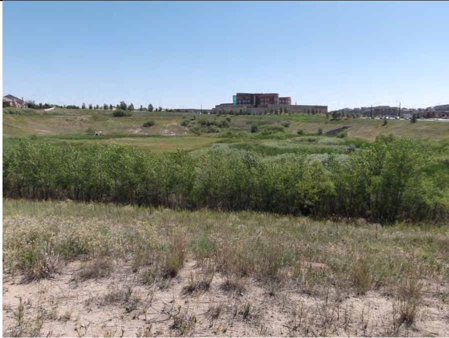
Photo 3. Looking east from RDF-C pond embankment showing existing constructed wetland along south side of pond (right half of pond bottom). Additional wetlands have established at other culvert inlets and groundwater seep points along the pond perimeter.
