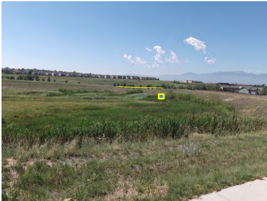
Photo 4. Looking south to pond outlet and spillway (highlighted in yellow) from RDF-C pond embankment.
