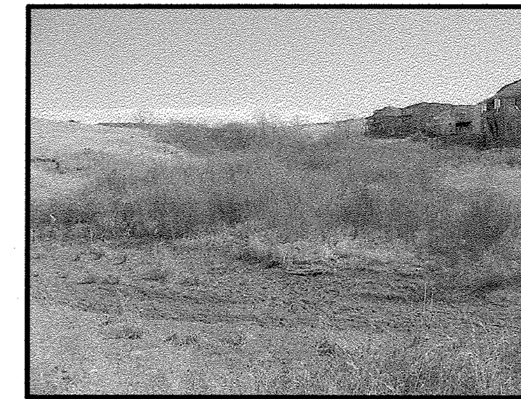
PHOTO #20 AT SPILLWAY OF EXISTING INLINE POND EAST OF DETENTION FACILITY 'E' LOOKING UPSTREAM
